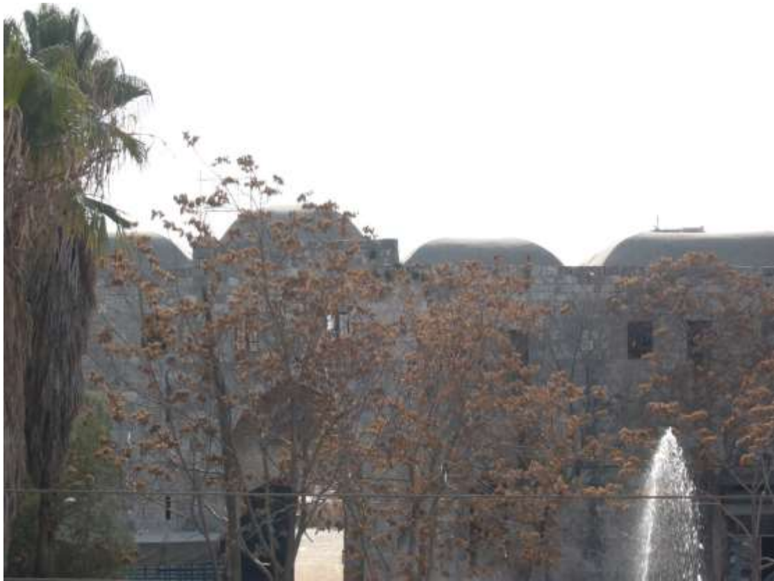
The northern façade of the building before the latest damage occurred
