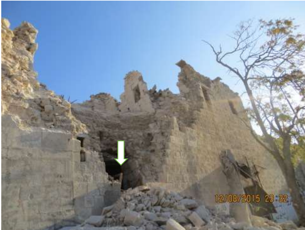
The northern façade of the Khan, after being hit with Airstrikes
