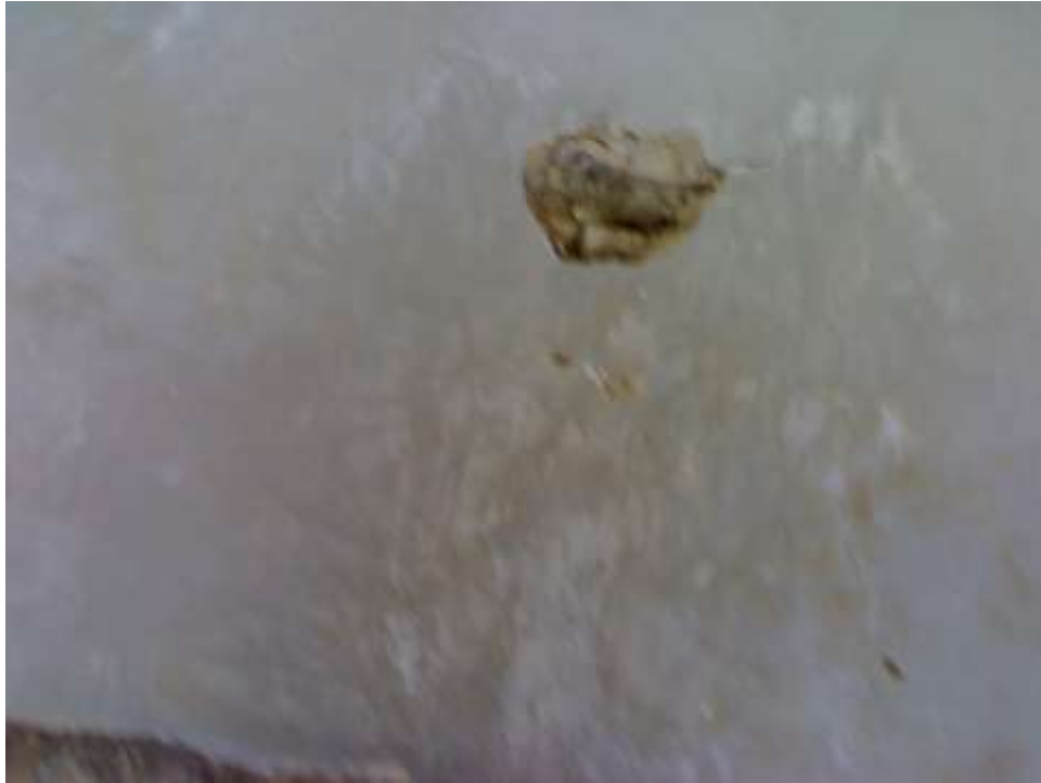
A partial opening in the roof
