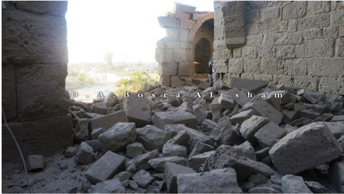
The arch connecting the second and fifth towers is destroyed.
