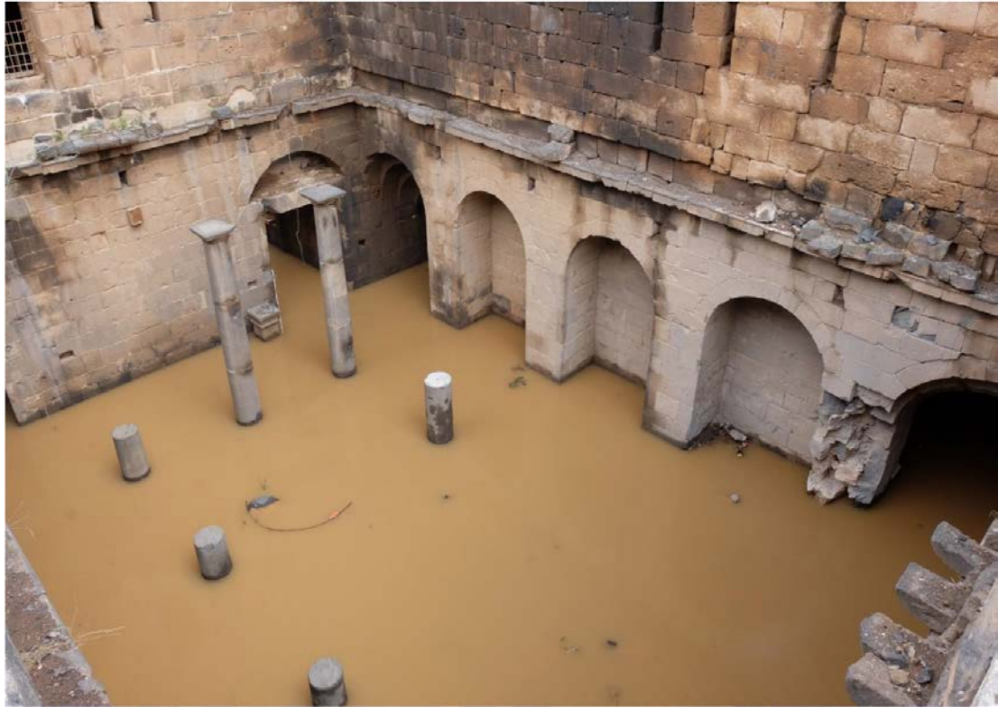
Another view of the west courtyard under water. Note the destruction caused by airstrikes.
