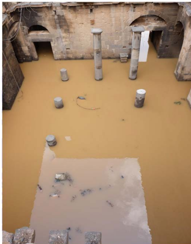
The west courtyard is under nearly 1.5m of water.
