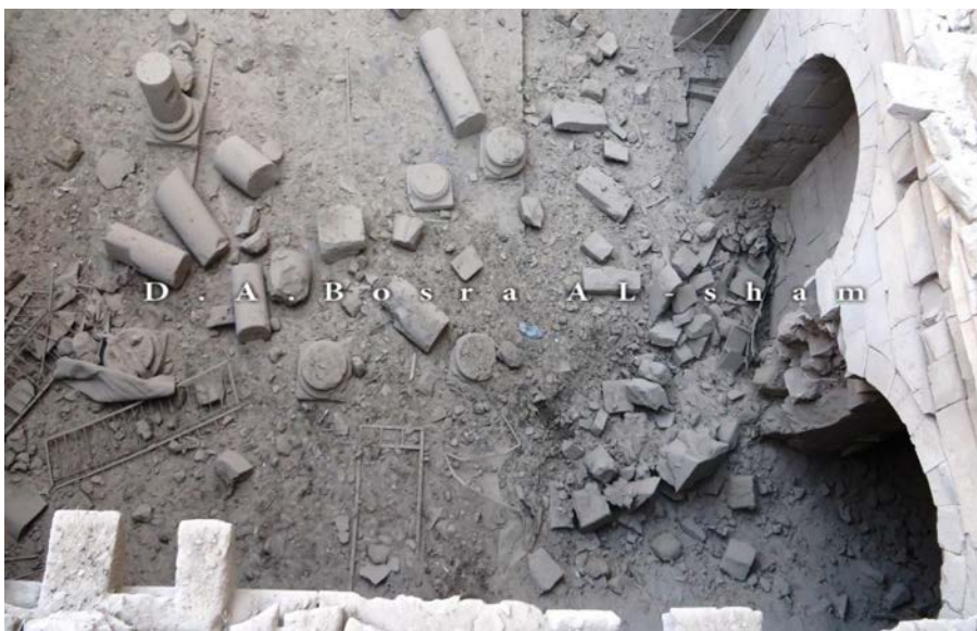
West courtyard after the airstrikes.
