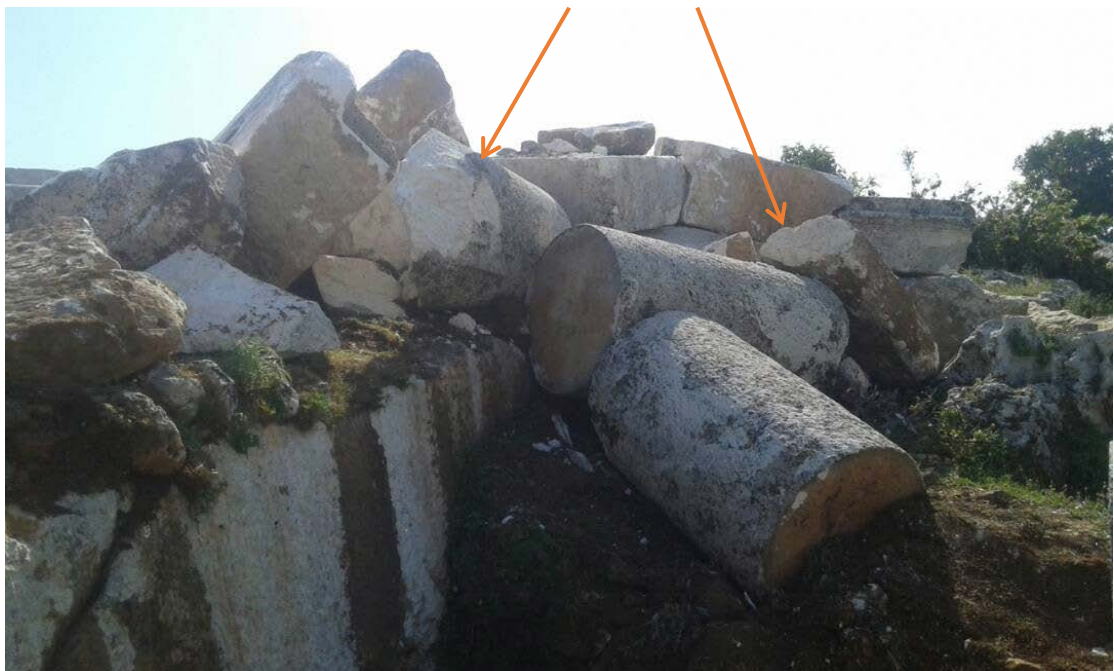
Stone masonry and columns damaged/broken and pushed to the side.
