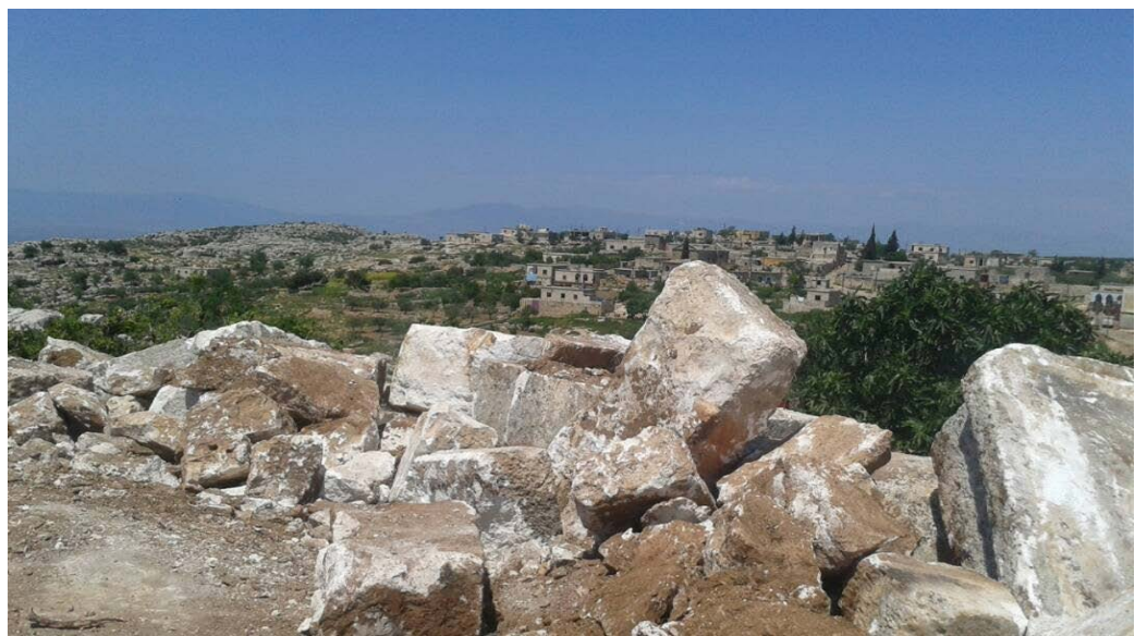
Damaged stone masonry
