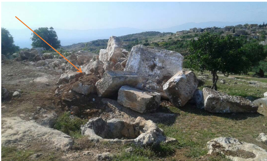
Destruction of the column with soil and stones moved by bulldozer
