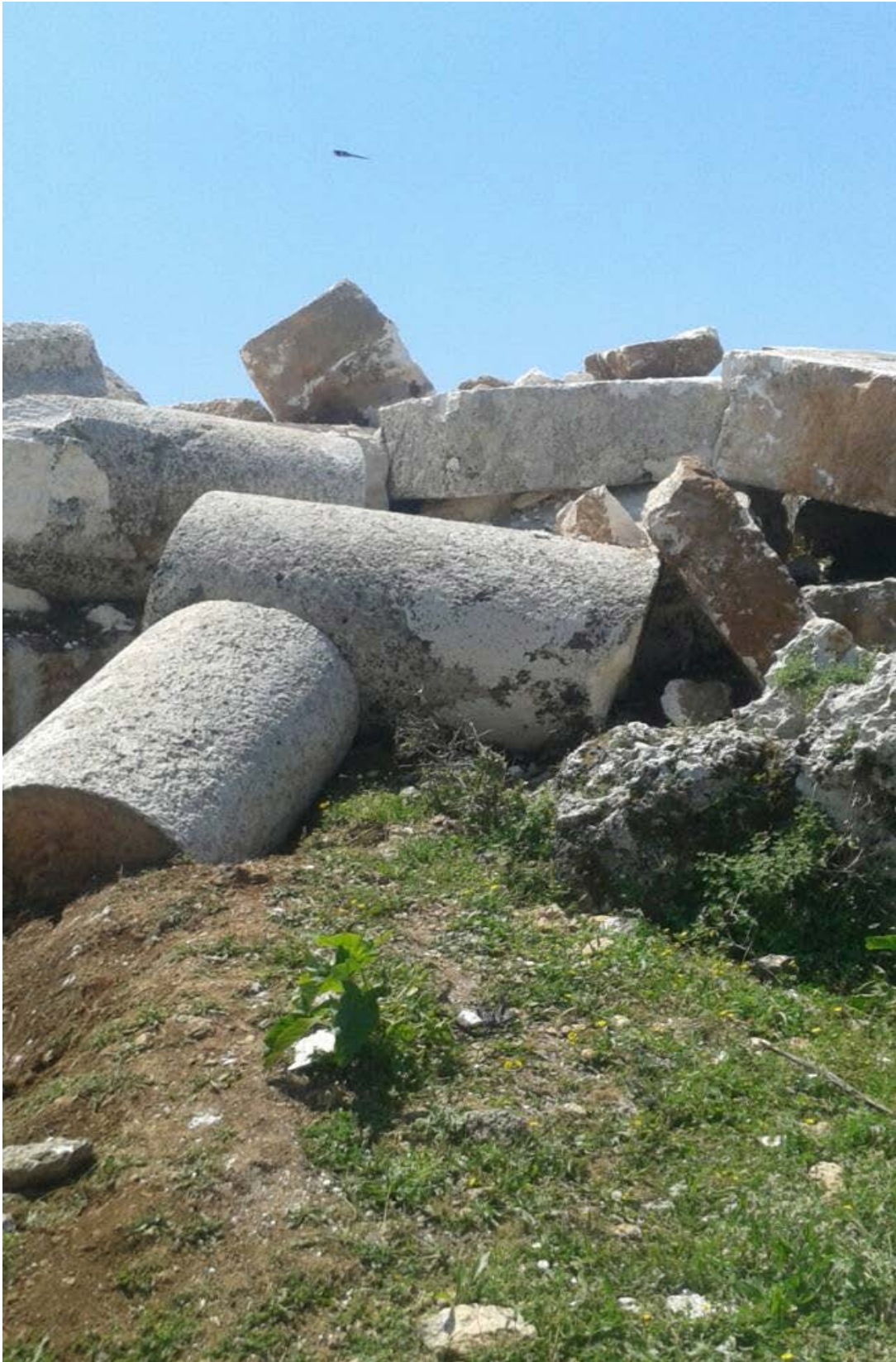
Damaged and smashed stone masonry and columns
