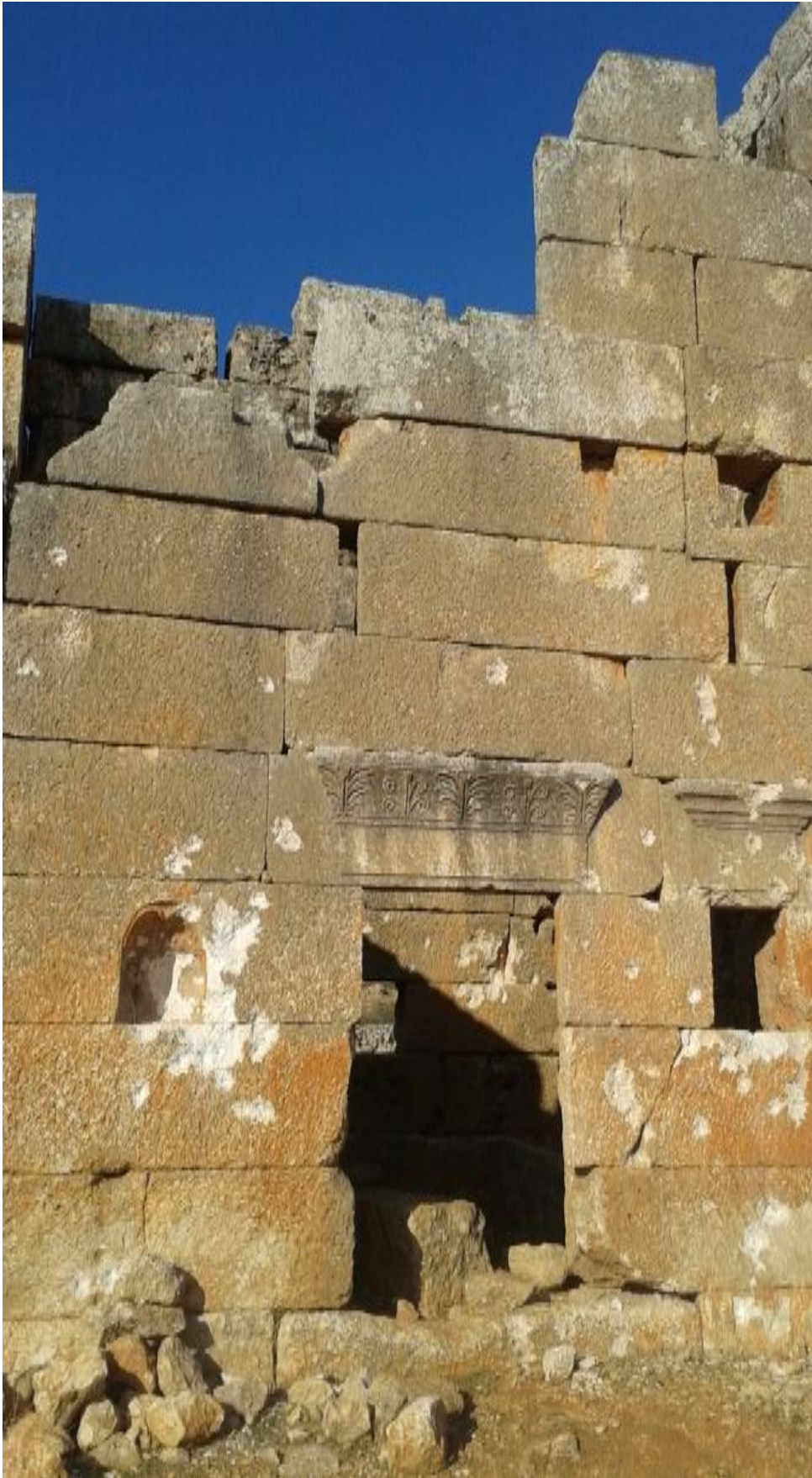
Photo showing bullet marks on the wall of a residential villa
