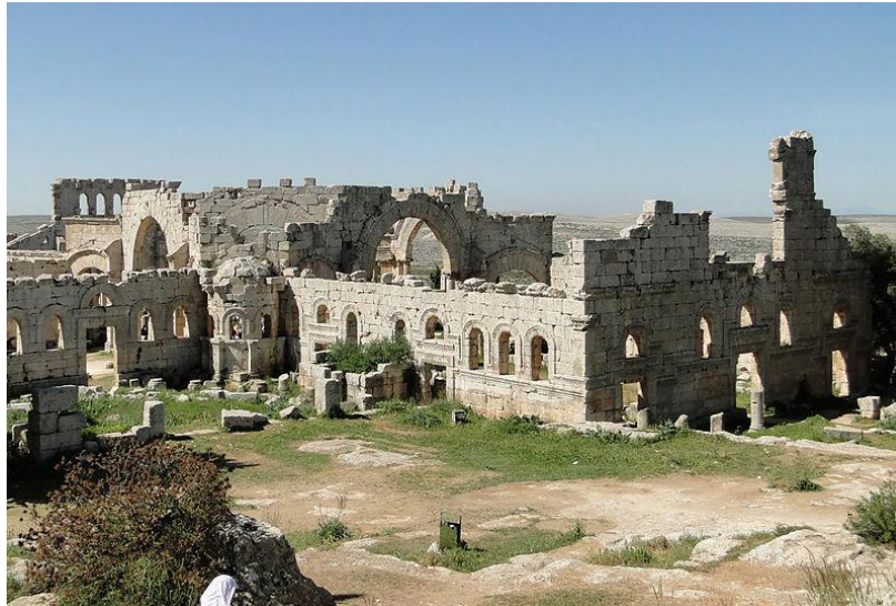
General view St. Simeon prior to the airstrike.
