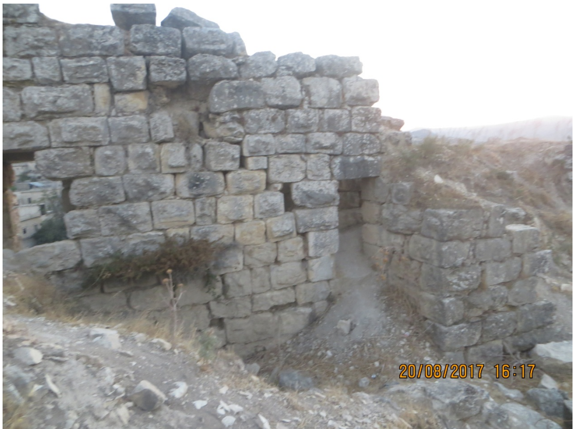
Collapse due to natural causes
