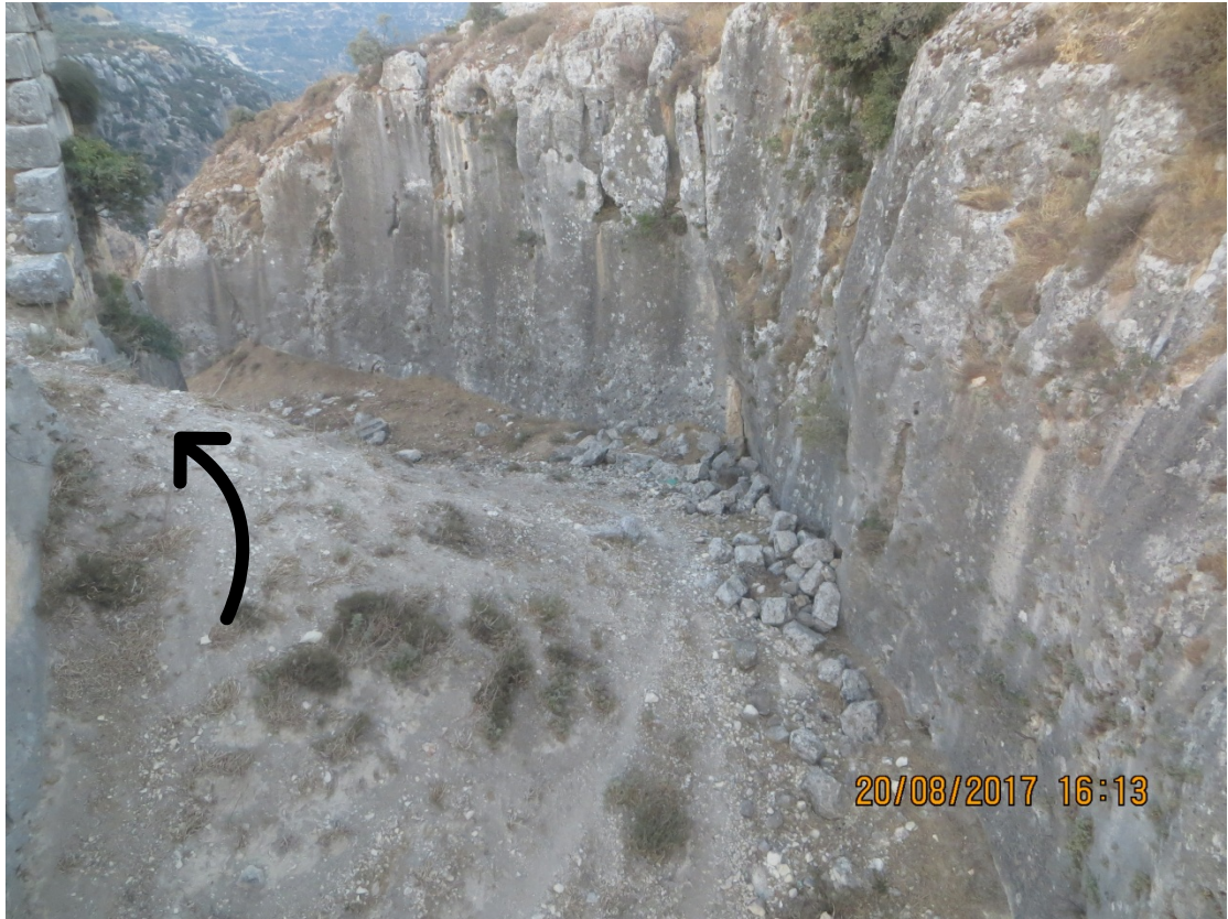
Collapse due to environmental /weathering
