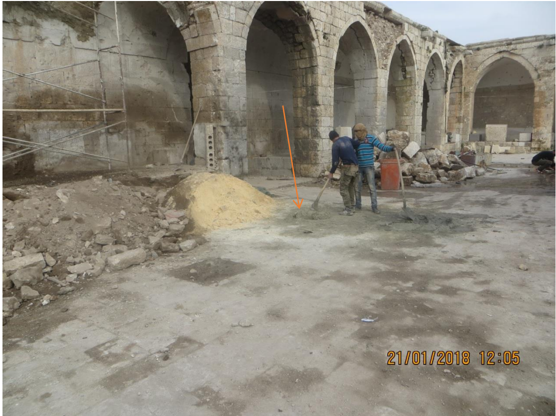
Preparing cement mix and applying it to damaged areas
