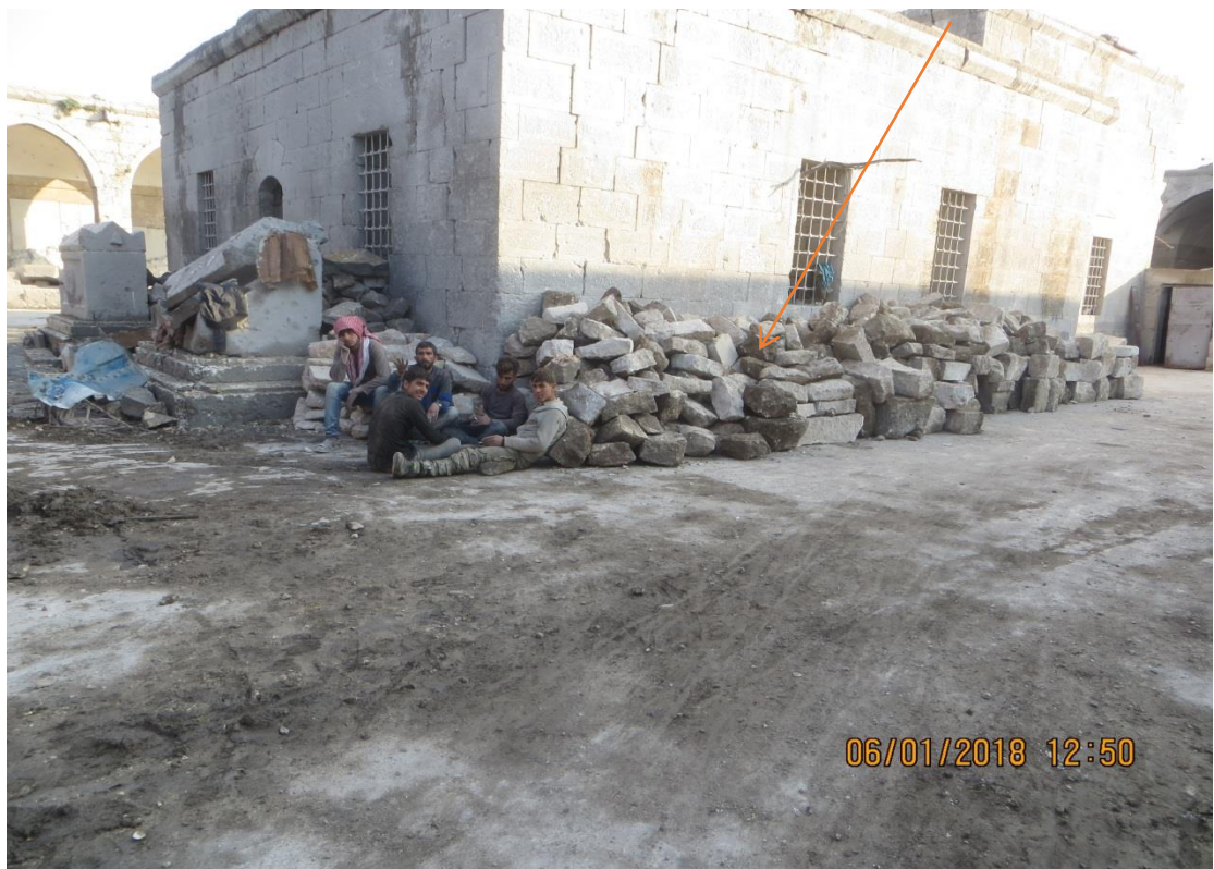
Gathering and sorting collapsed masonry
