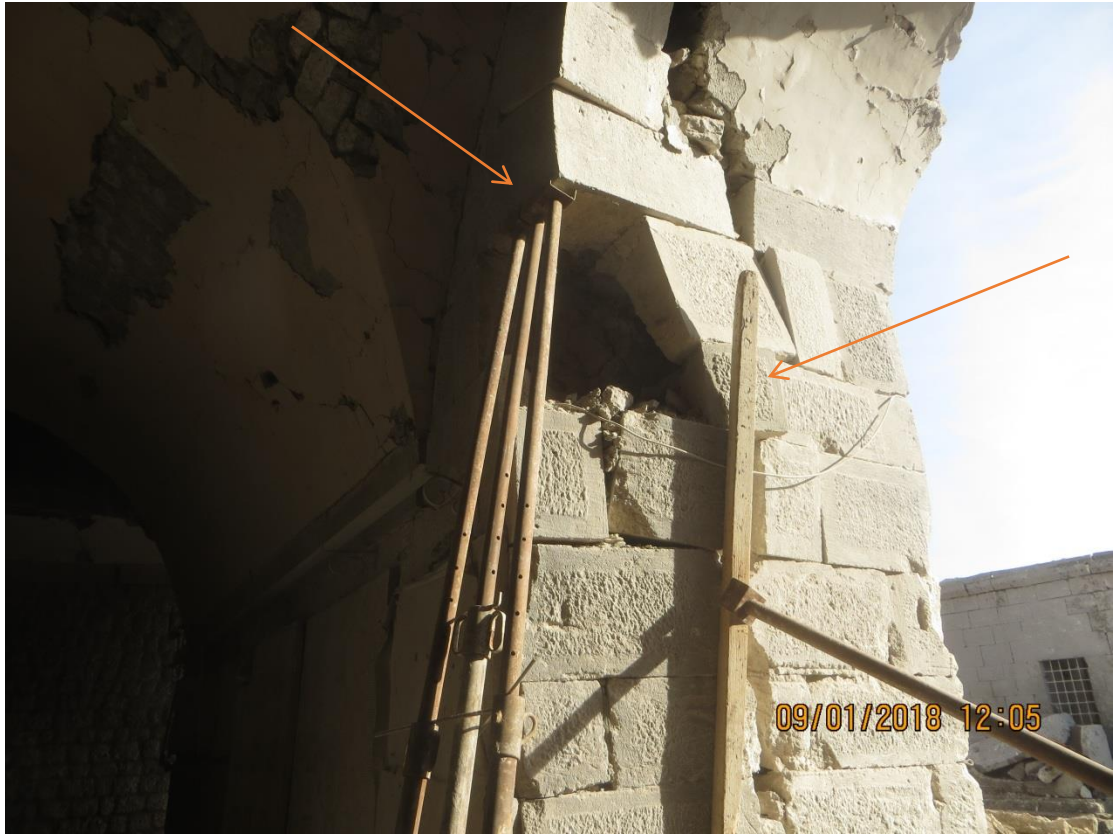
Stabilizing damaged areas using wooden beams and scaffolding
