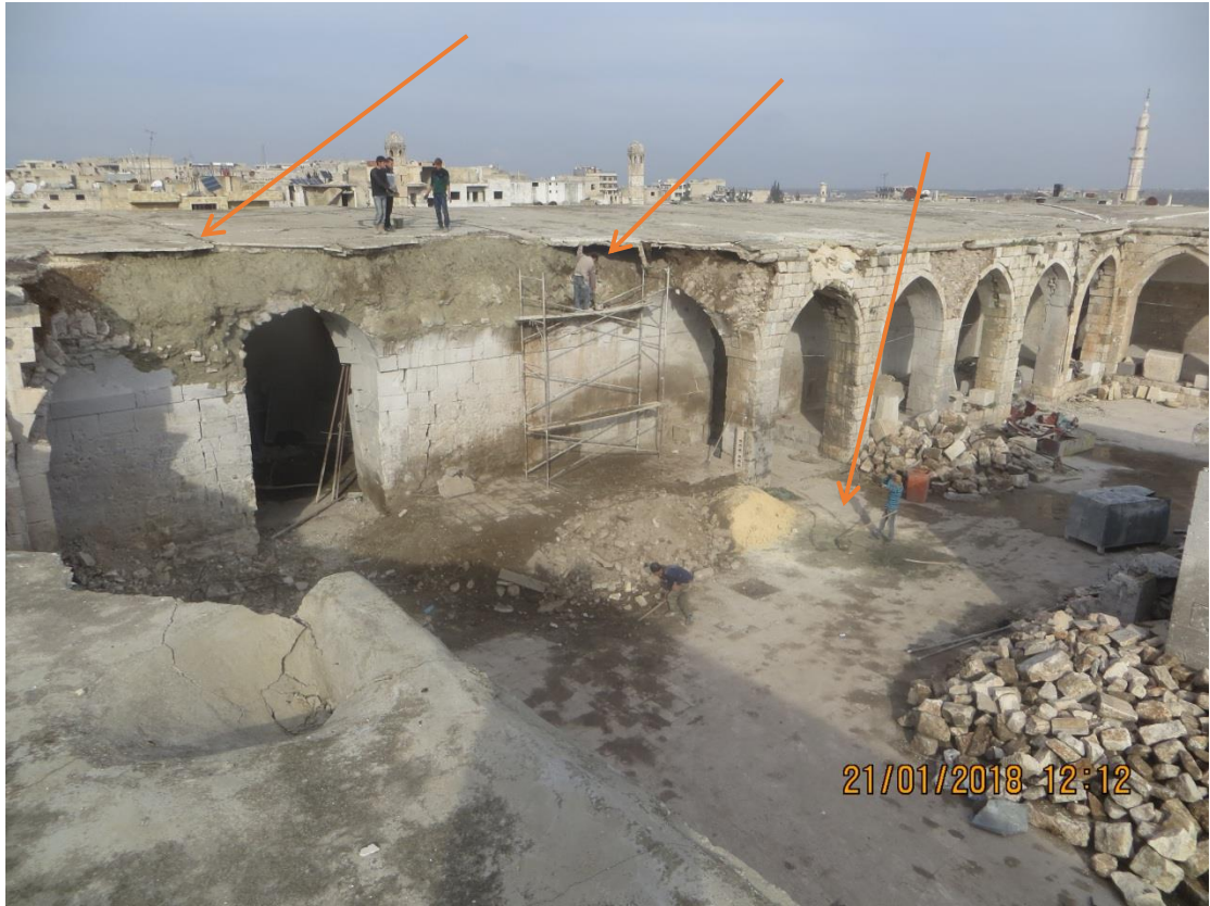
Ongoing repair to prevent deterioration of damaged areas from environmental conditions
