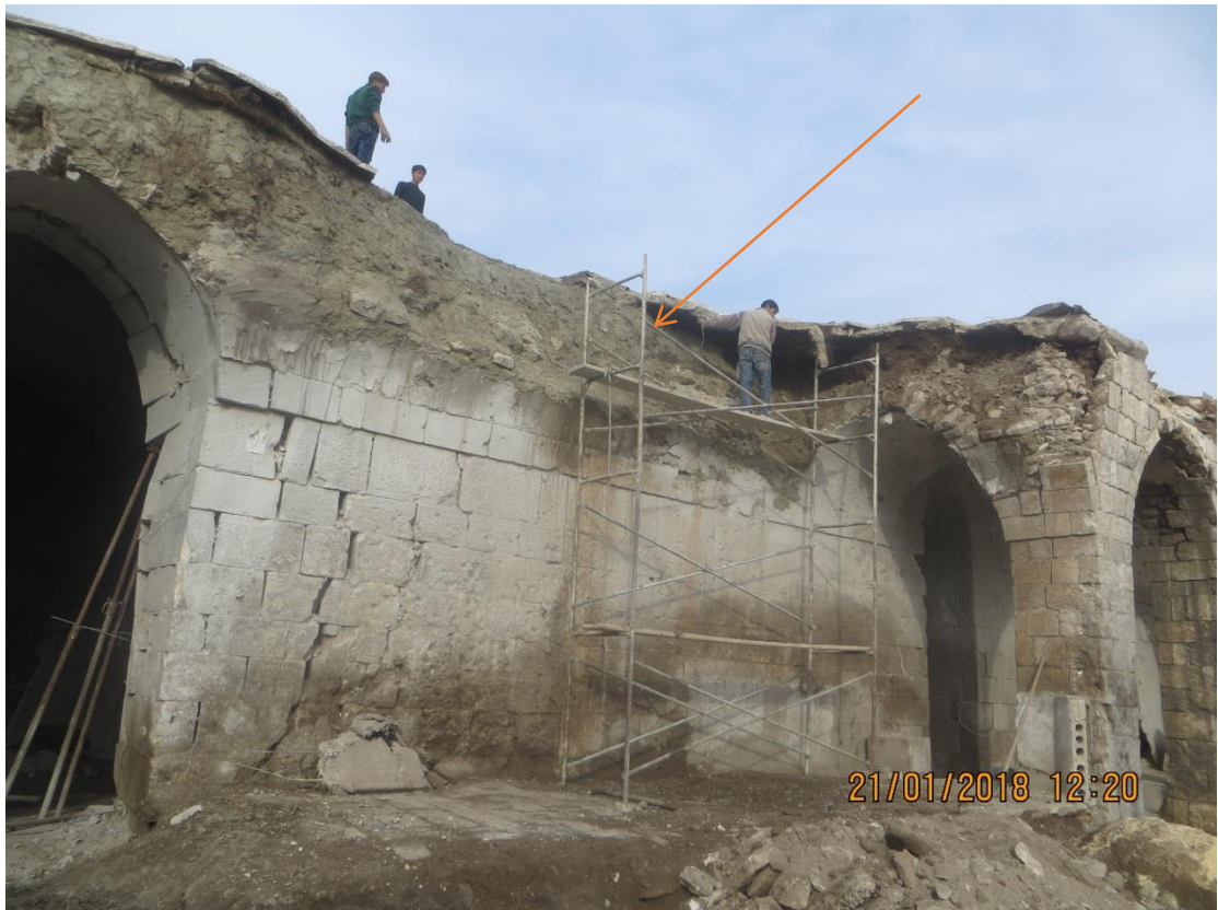
Preparing cement mix and applying it to damaged areas
