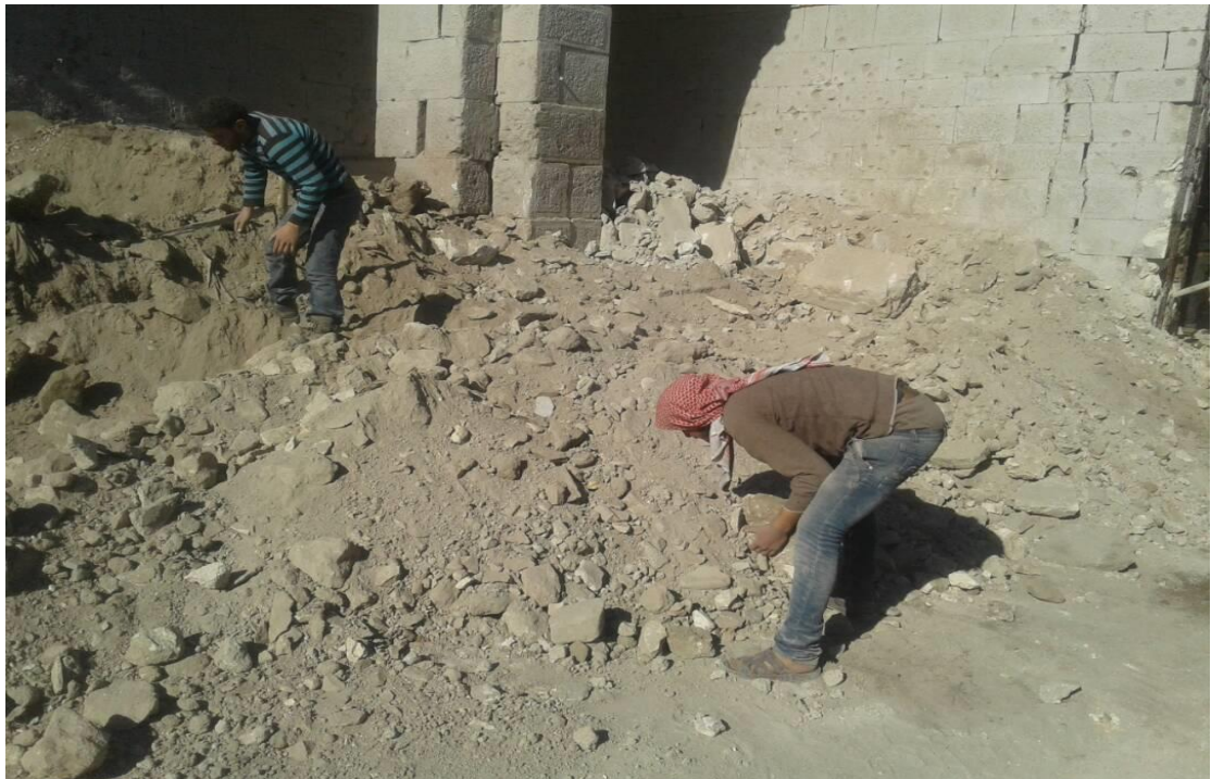
Digging out the rubble and collecting fallen masonry
