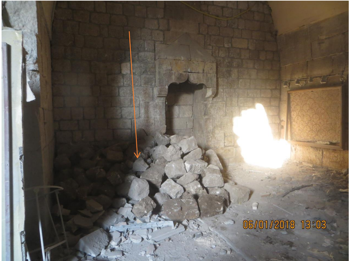
Gathering collapsed masonry
