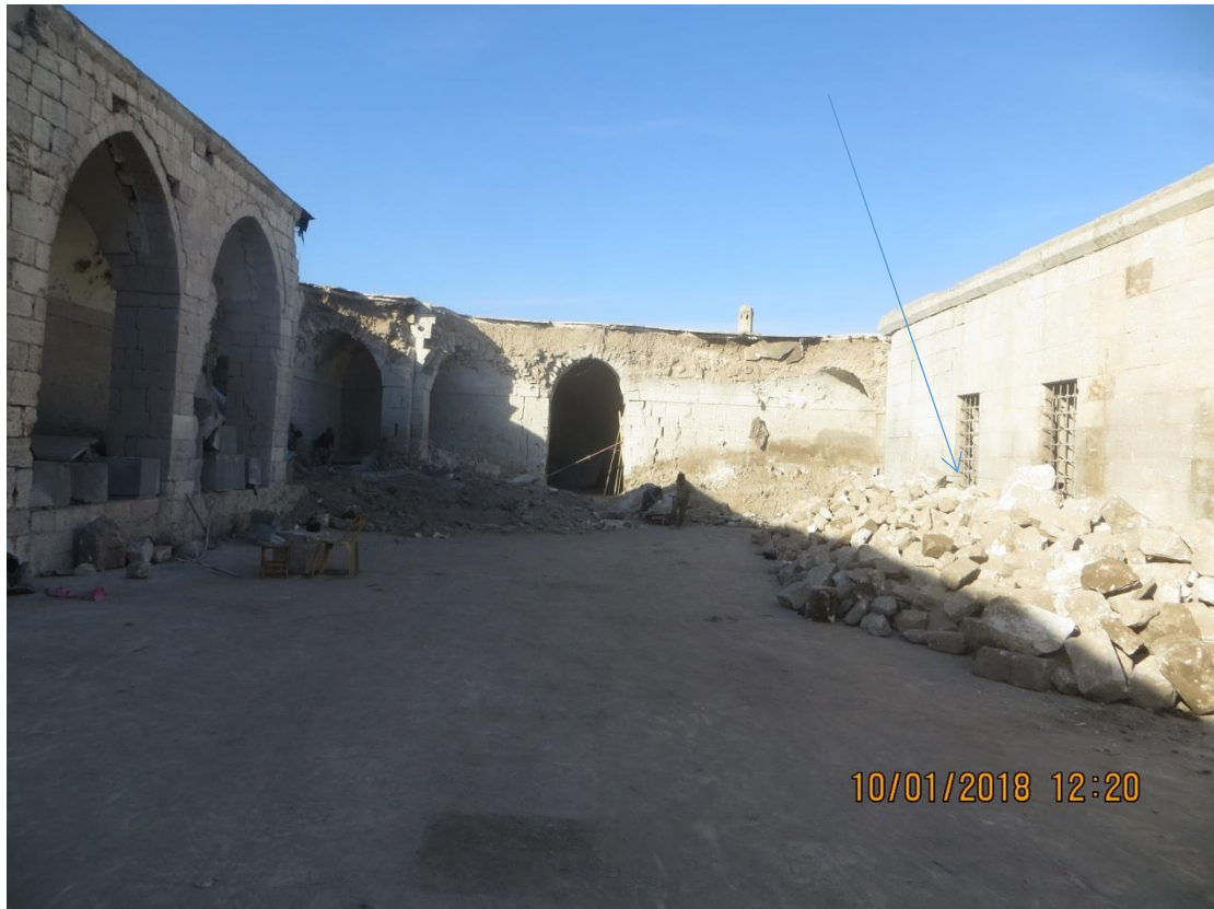
Gathered masonry from the north and west façade
