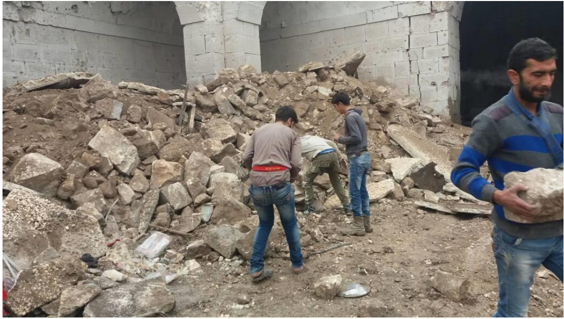
Digging out the rubble and collecting fallen masonry
