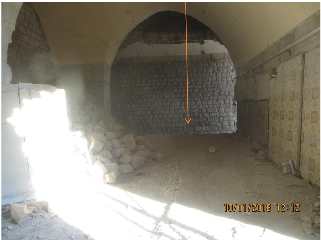
After collapsed rubble removal
