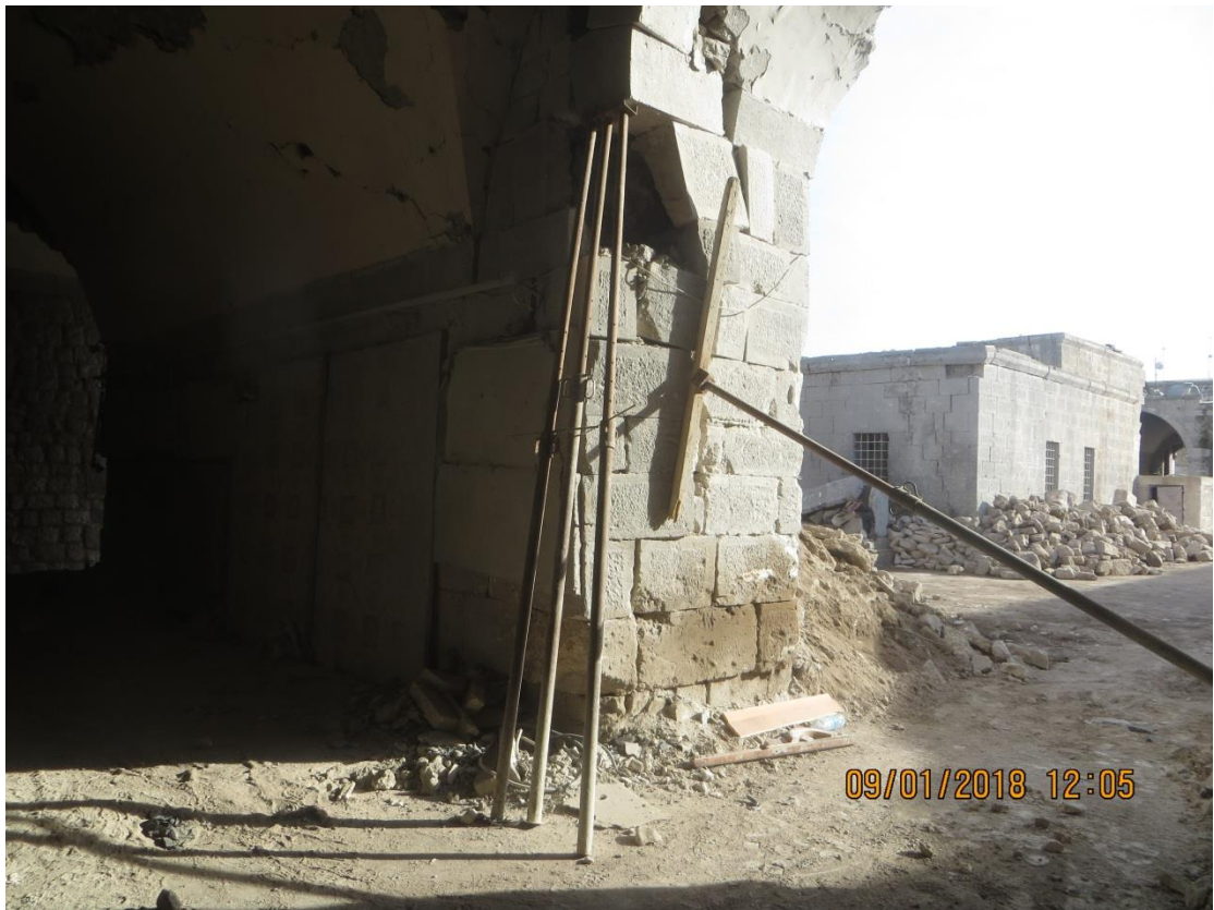
Stabilizing damaged wall area supporting arch
