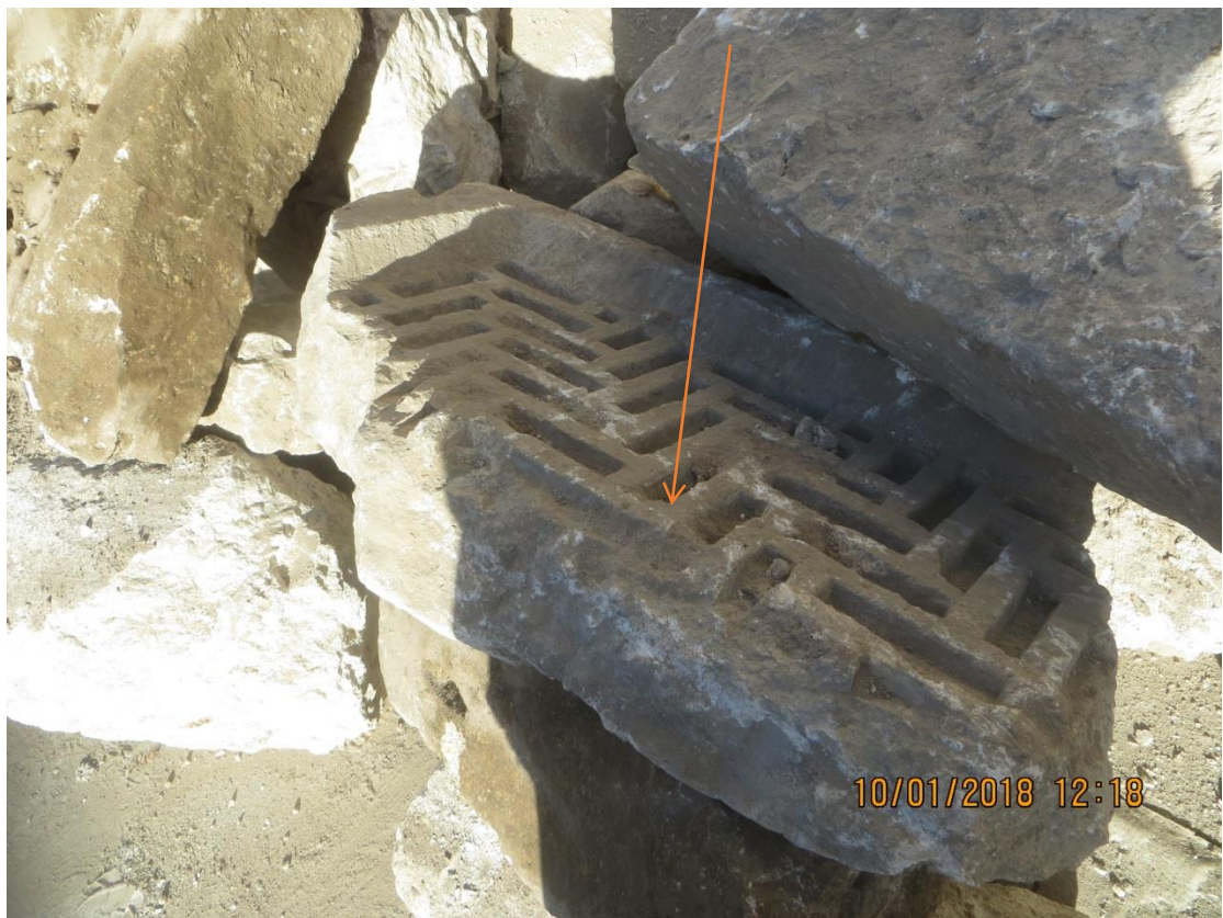
Masonry from the damaged tomb facade
