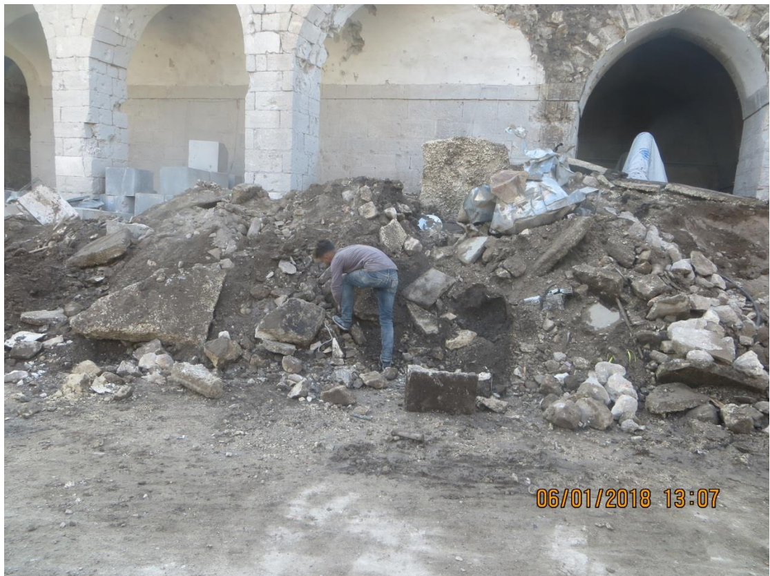
Digging out the rubble and collecting fallen masonry
