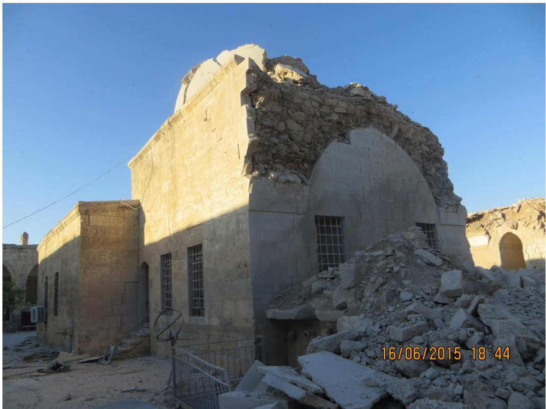
The southwest corner of the mosque
