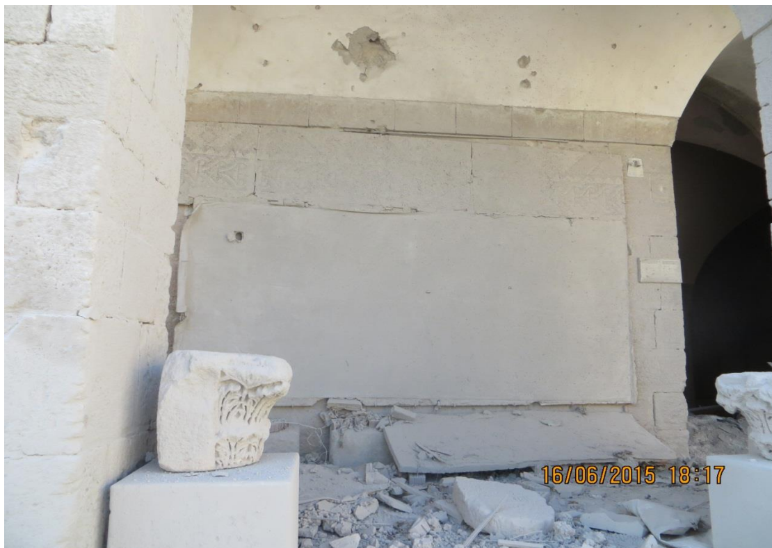
Mosaic panel covered with a layer of glue and cloth exposed after the fall of the sand bags due to the blast.
