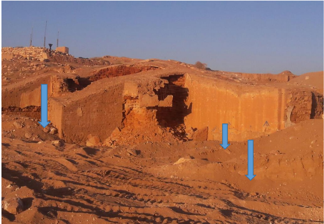
Arrows pointing damage caused by the airstrikes and their aftermath
