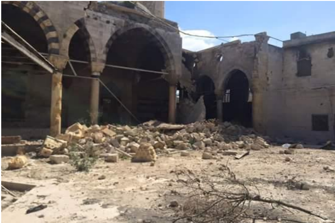
Damage caused by an explosive barrel bomb dropped by Syrian regime
