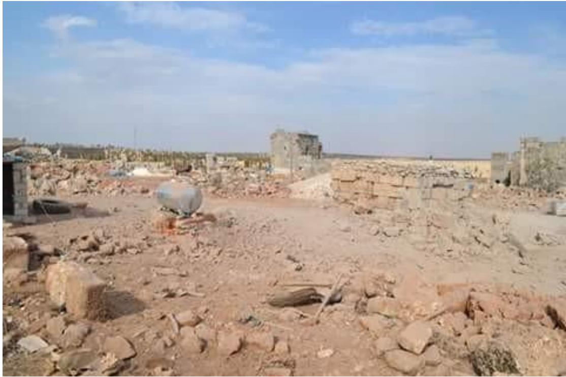
Destruction caused by recent Russian bombing (eastern side)
