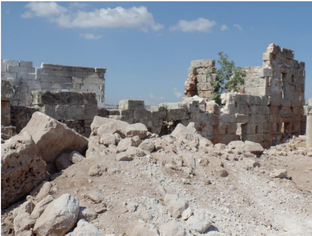
Collapse of the entire archaeological building
