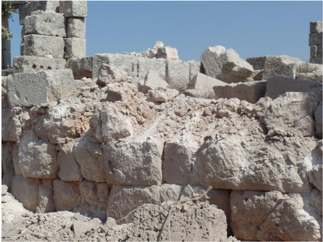
Collapse of the entire archaeological building
