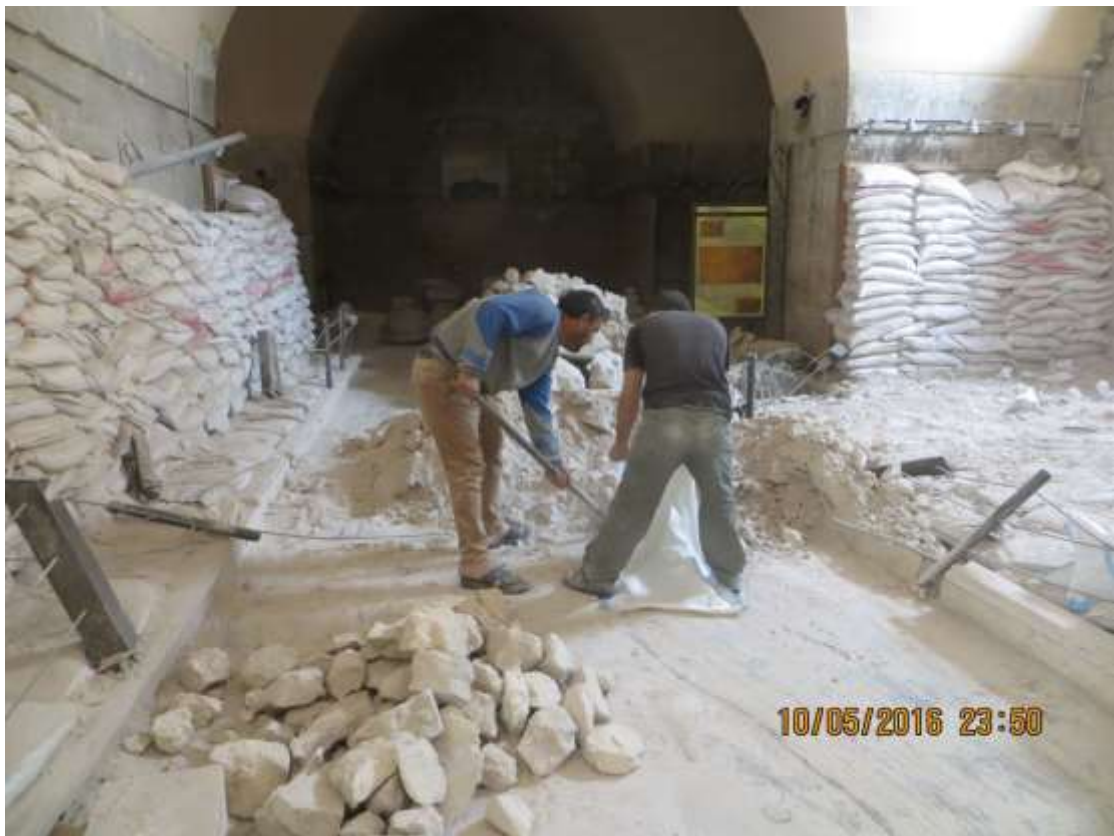
Filling up new sandbags
