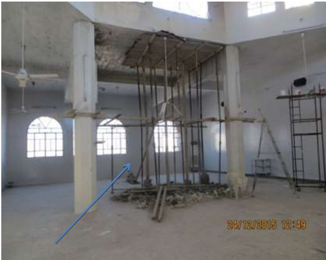
Scaffold in place to shore up damaged section of the building
