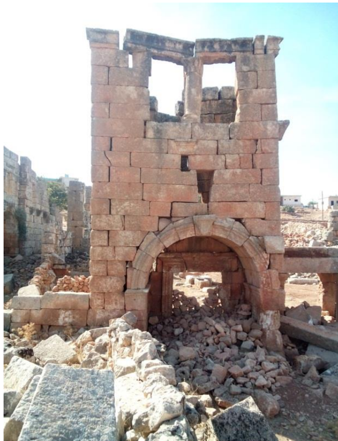
Damage caused by neglect
