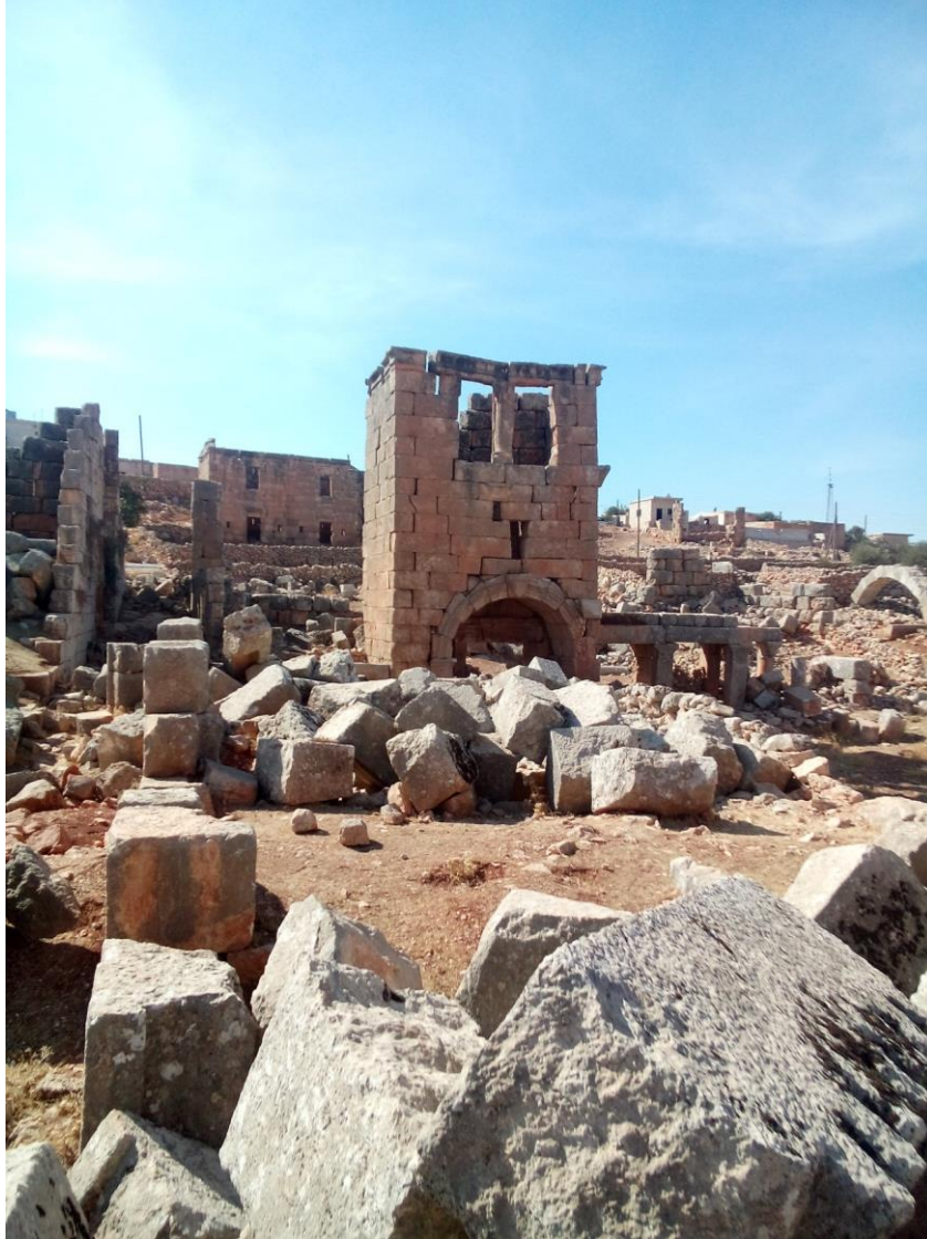
Damage due to weathering and neglect
