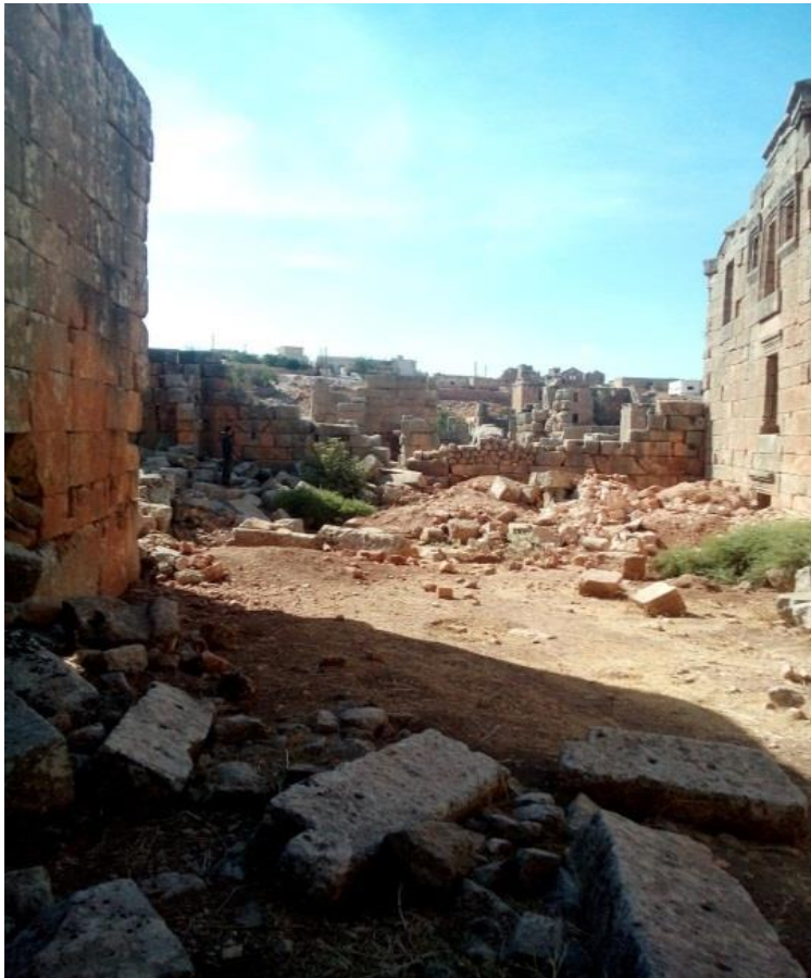
Damage due overgrowth of plants
