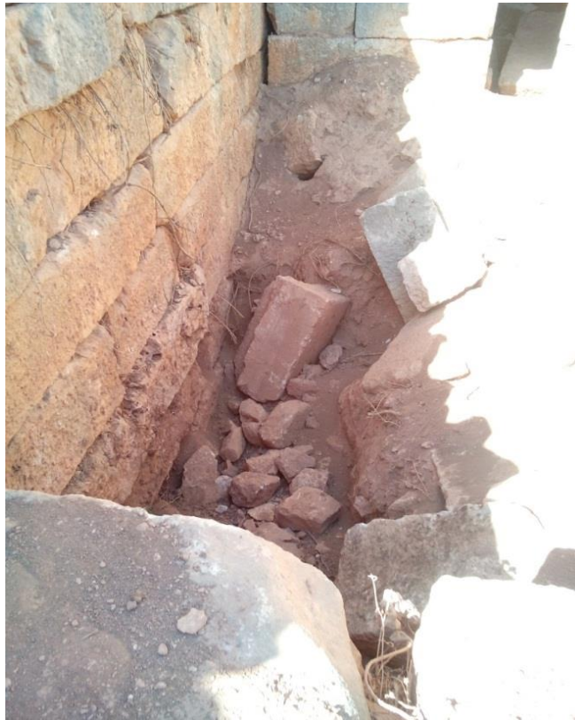
Illicit digging near the walls
