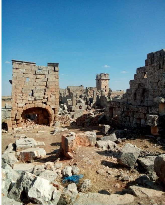
Damage caused by neglect
