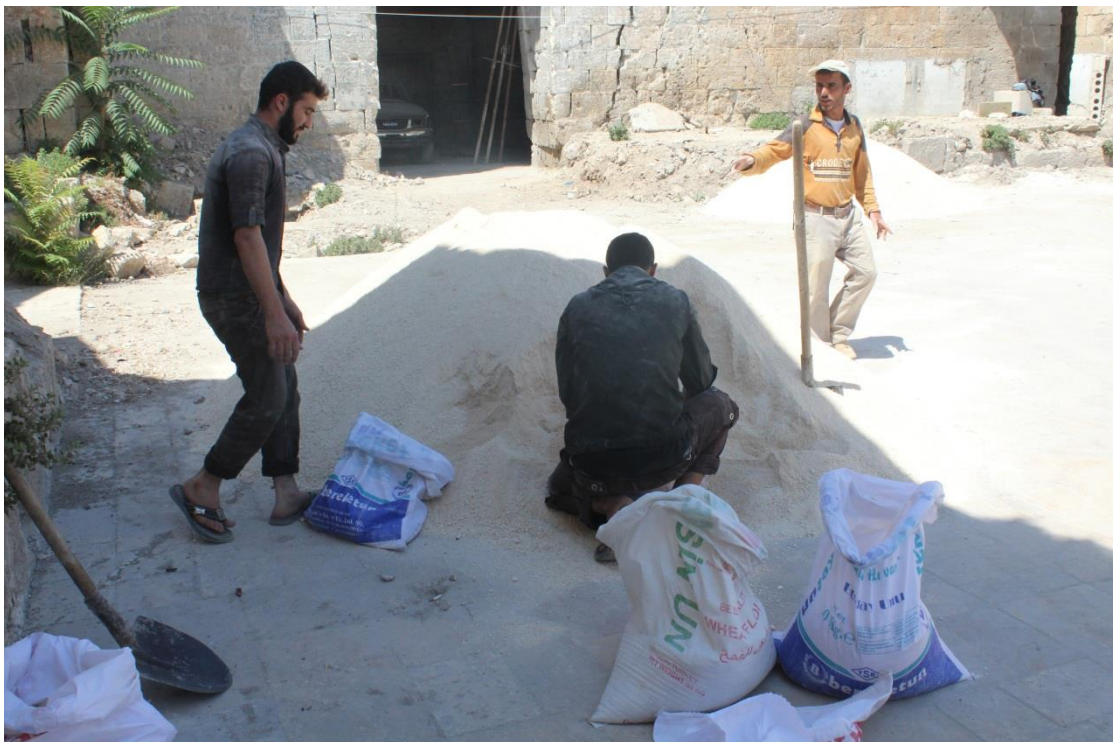
Filling up sandbags for protecting mosaics
