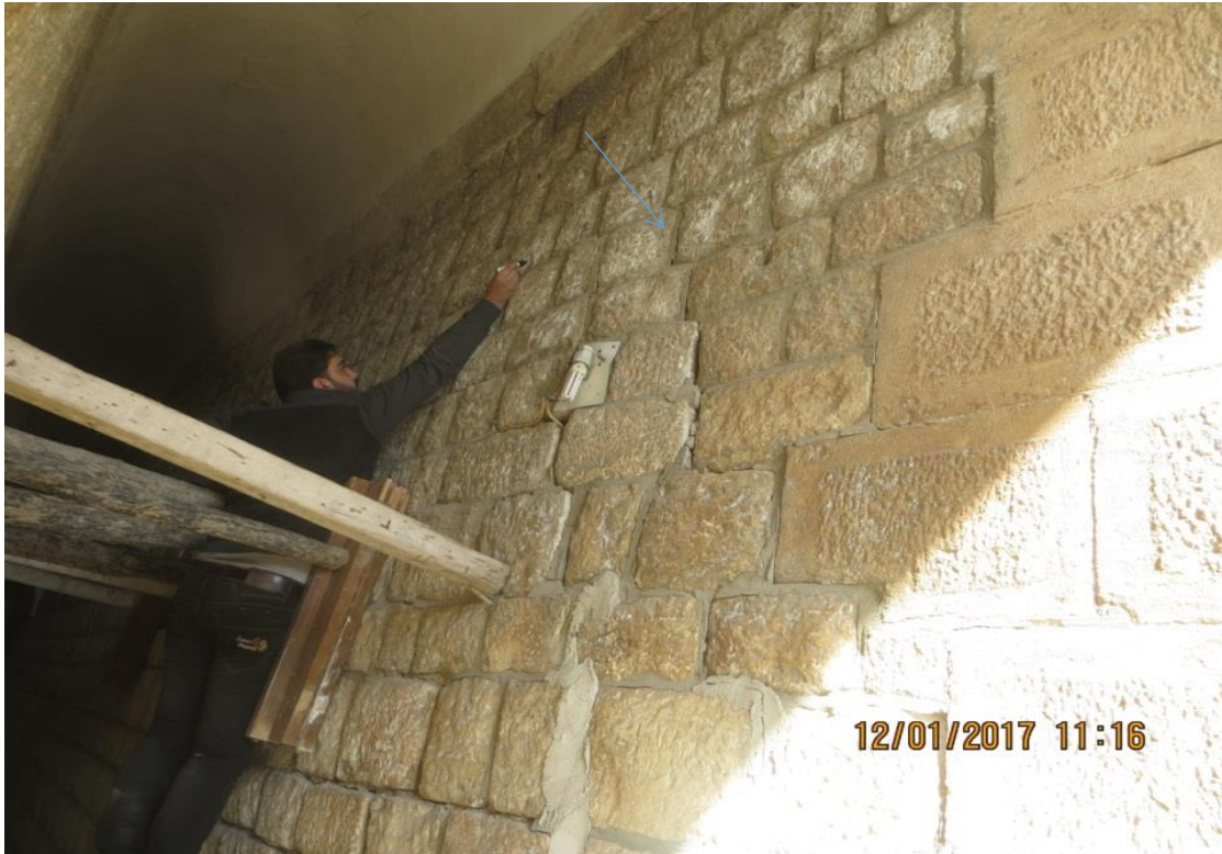
Numbering bricks where deviation begins
