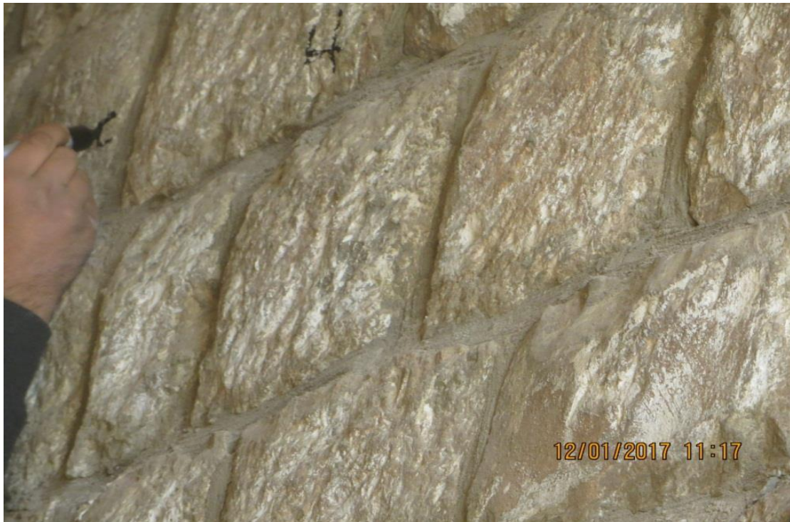
Numbering bricks where deviation begins
