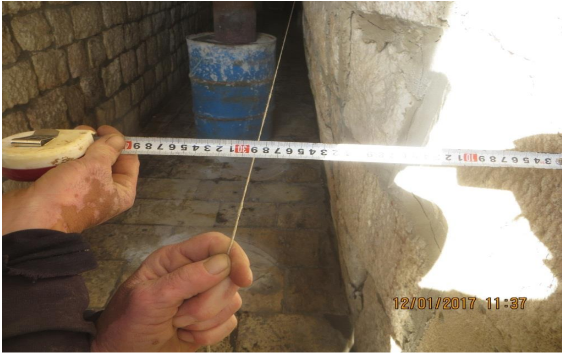
Measuring wall deviation
