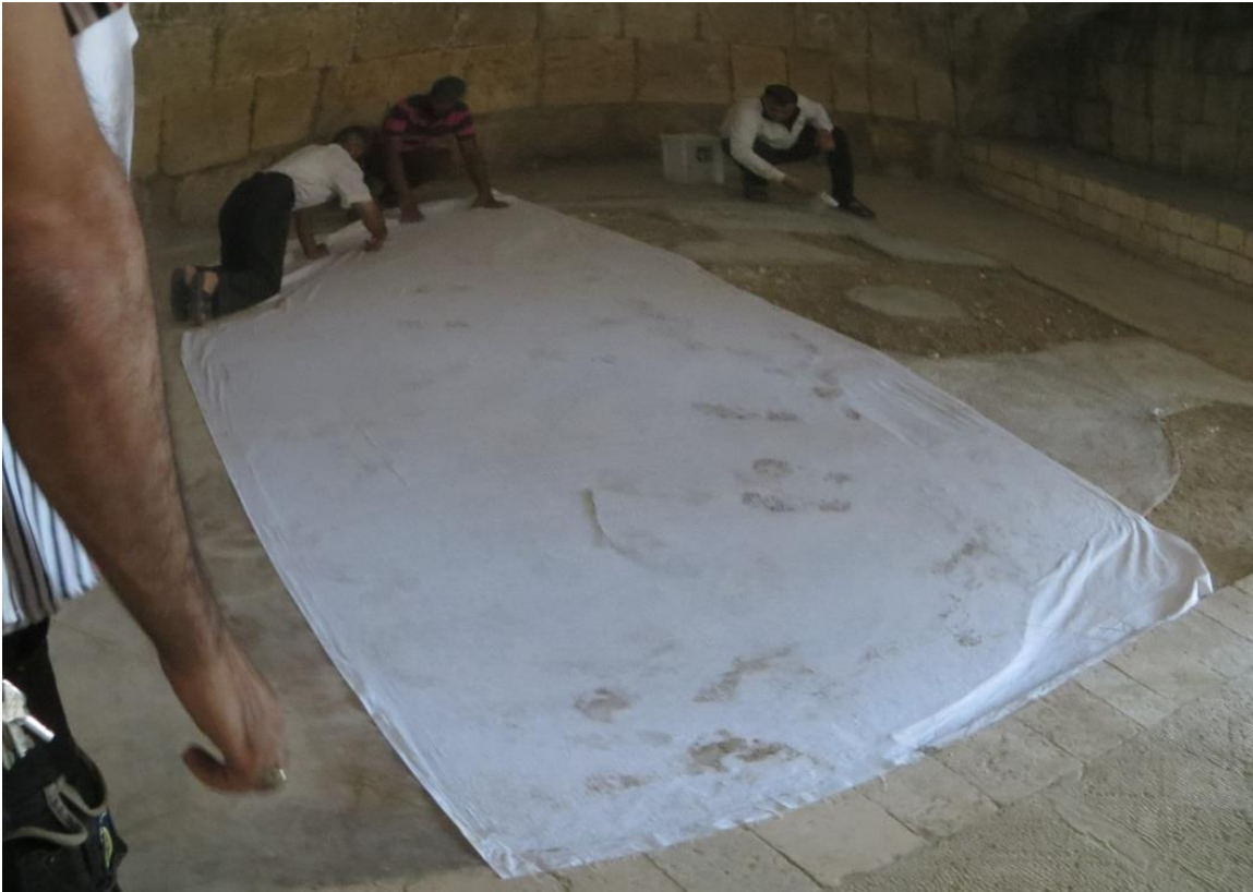
Gluing cotton sheets onto the mosaic floors
