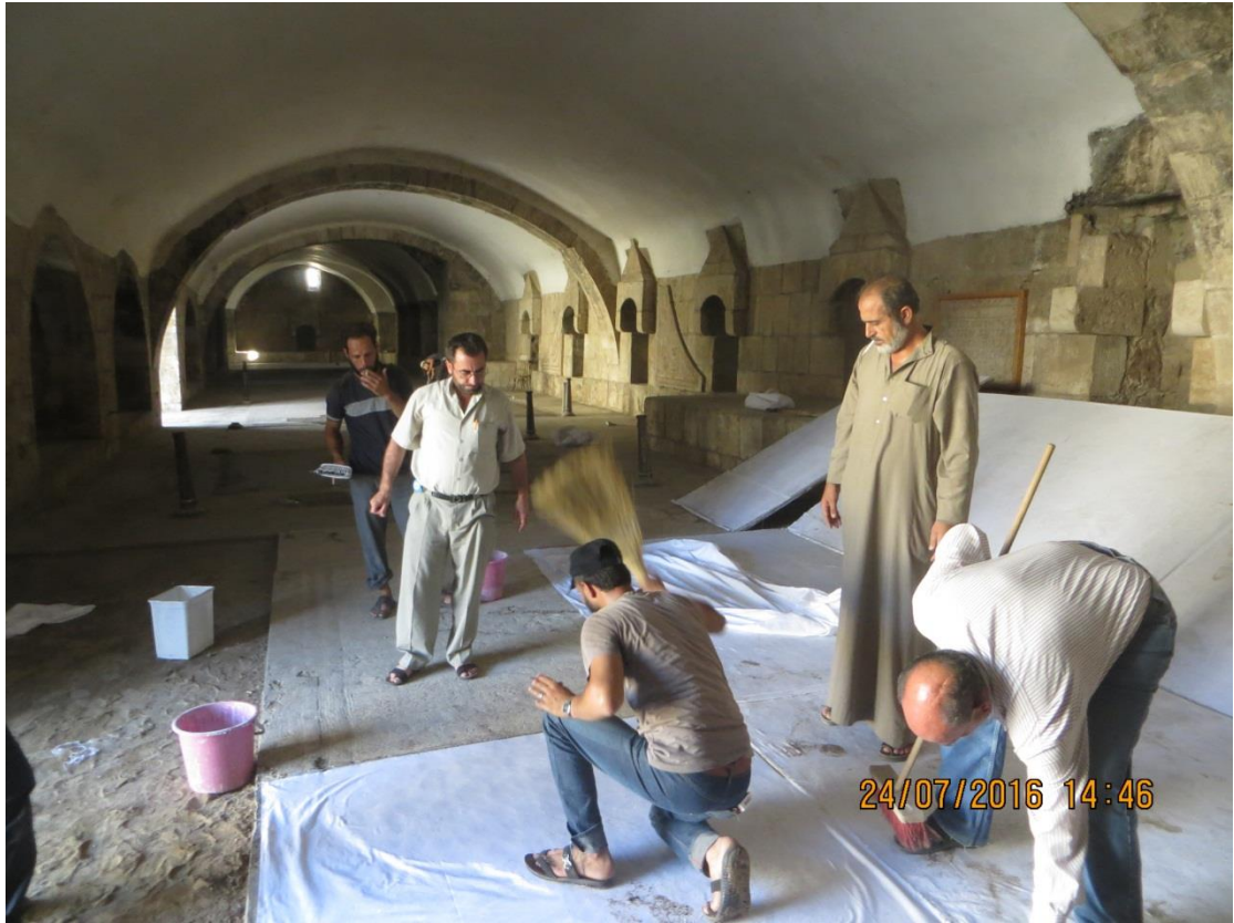
Gluing cotton sheets onto the mosaic floors
