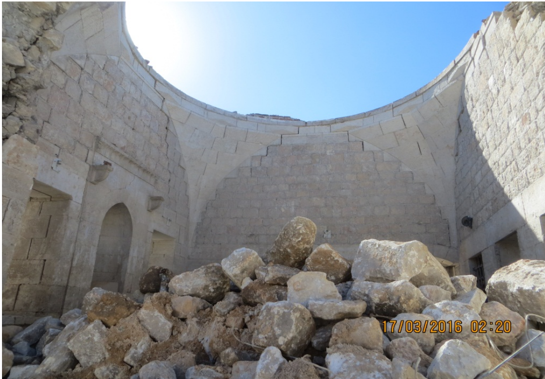
View from inside the mosque looking up at where the dome used to be
