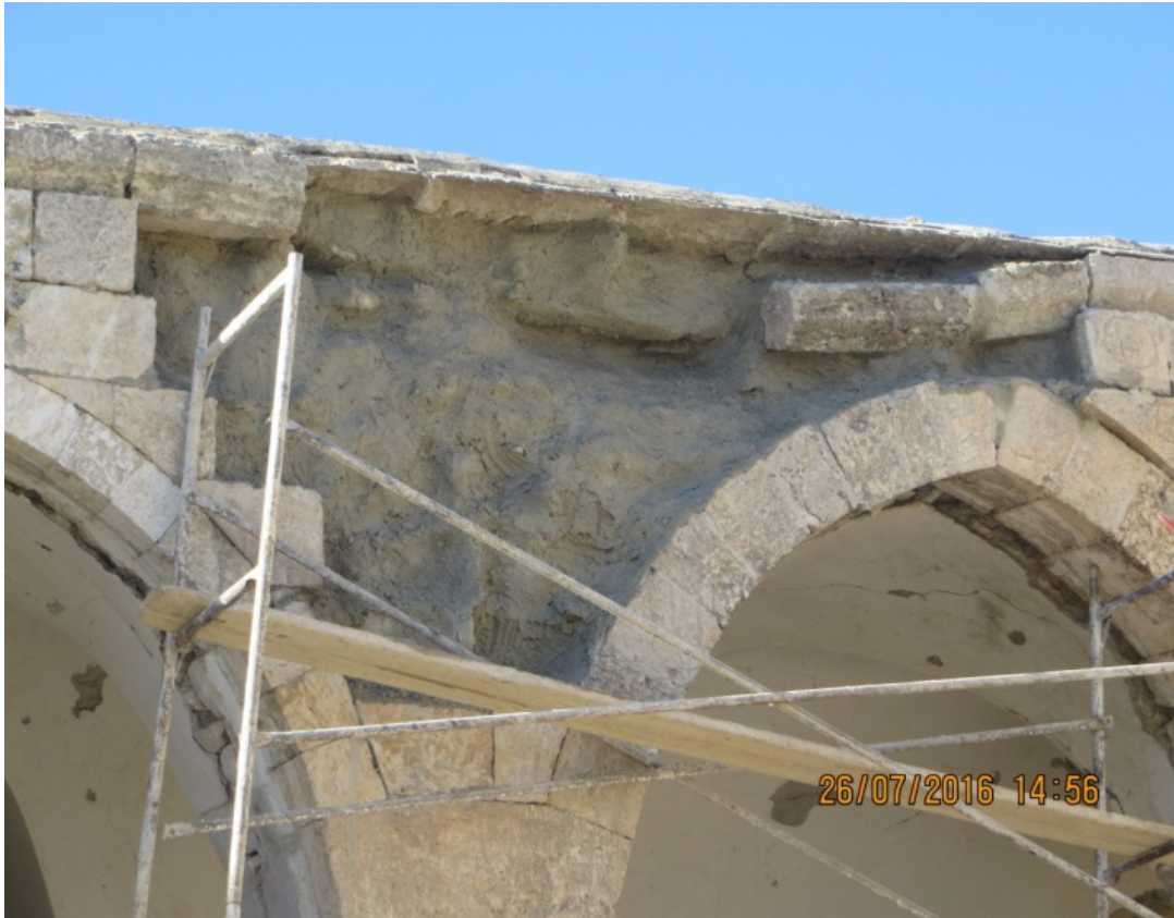
Cement mortar patch
