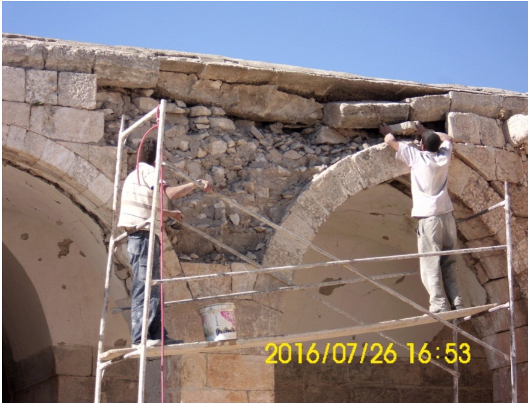
Patching the exposed damage area around the supporting arch with cement mortar
