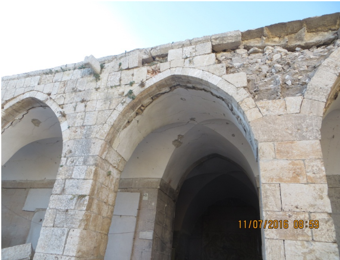
Damage to the arches and the ceiling in the east gallery
