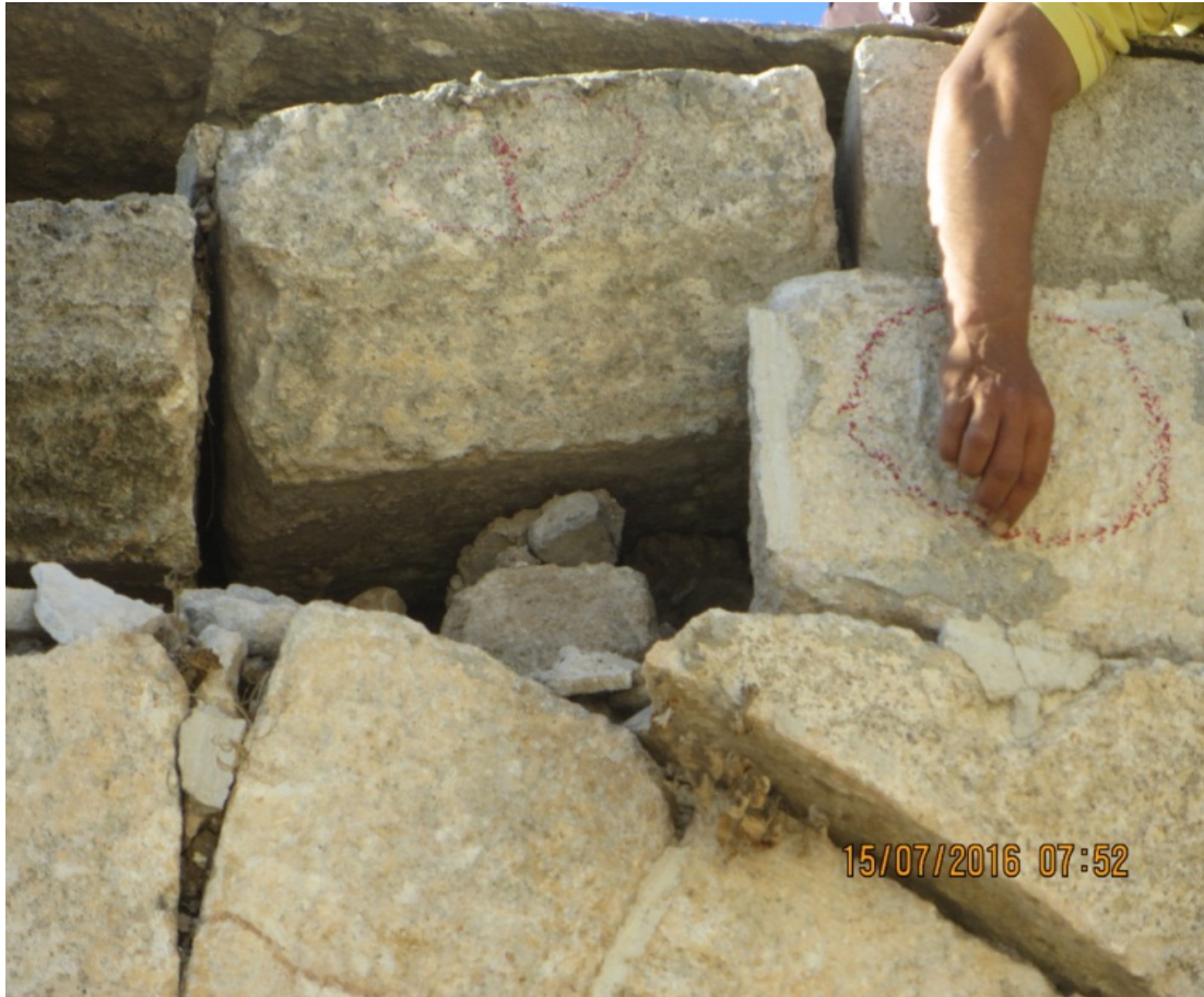
Labelling weak and unstable stone masonry for removal (continued)
