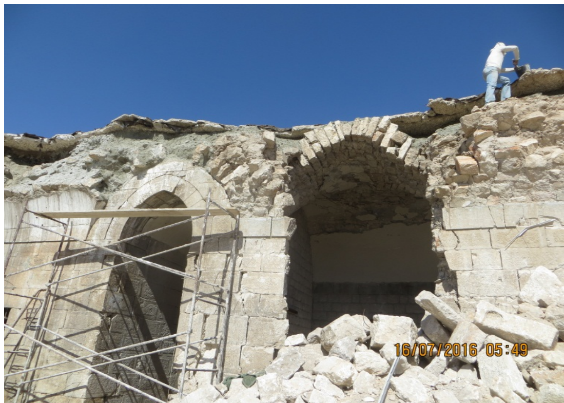
Loose masonry and exposed roof/wall fill
