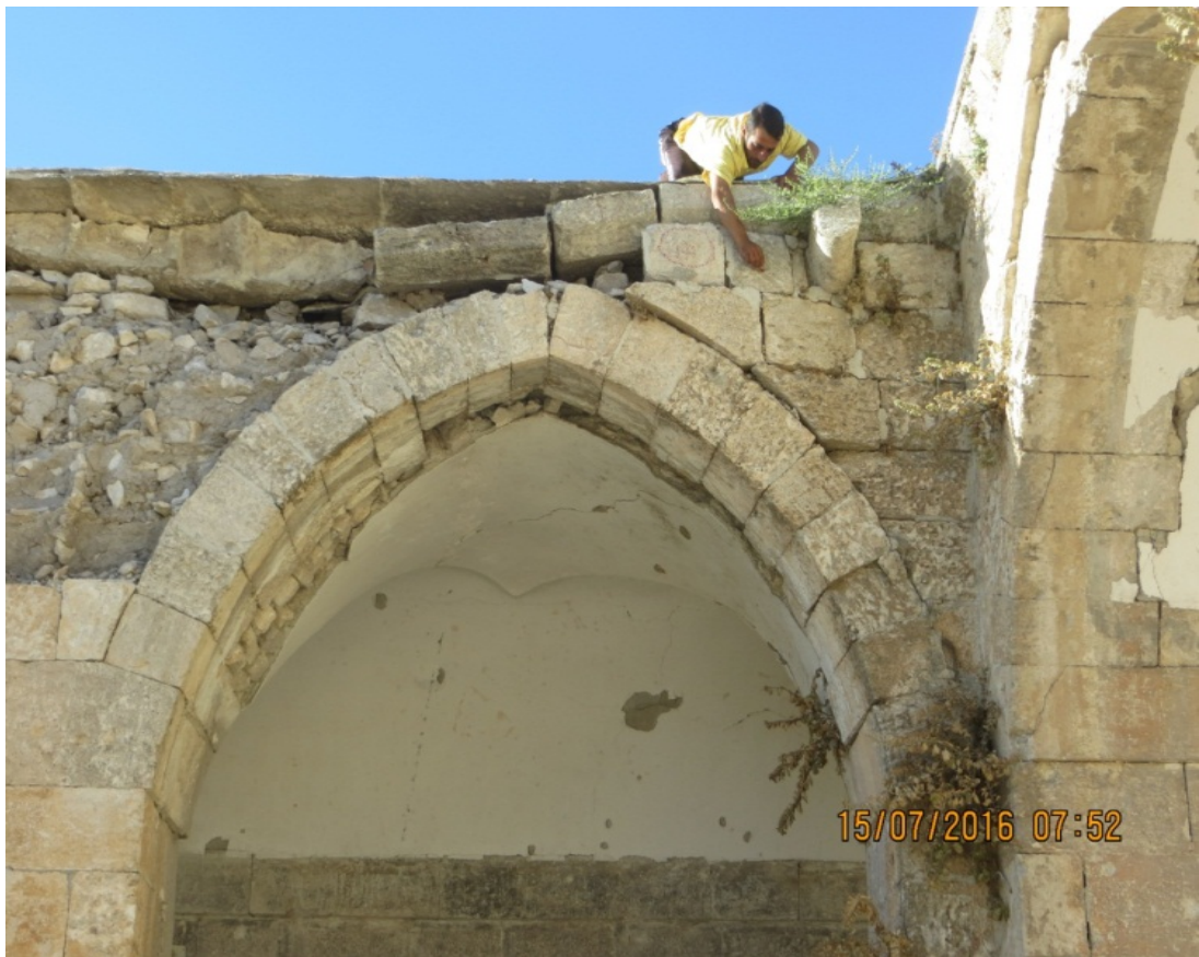
Labelling weak and unstable stone masonry for removal
