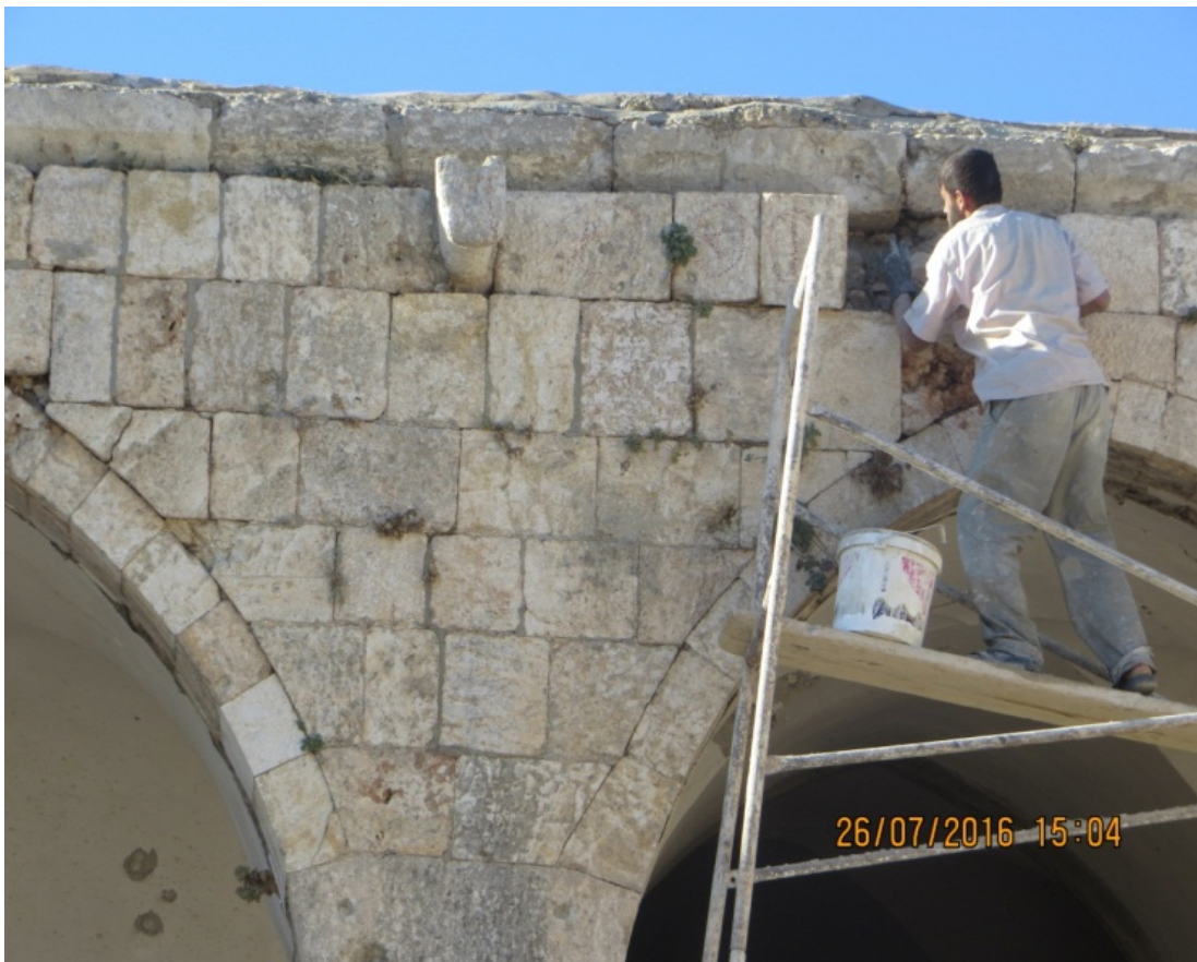
Cement mortar patch
