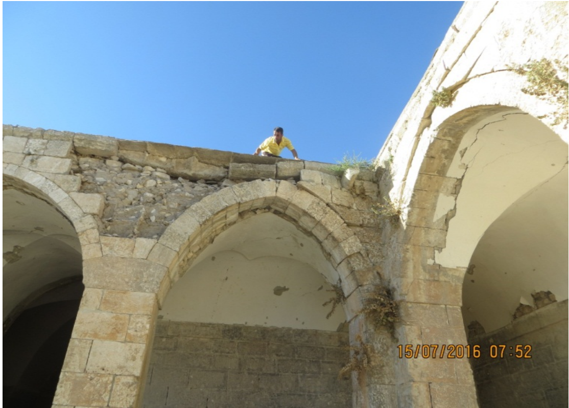
Labelling weak and unstable stone masonry for removal
