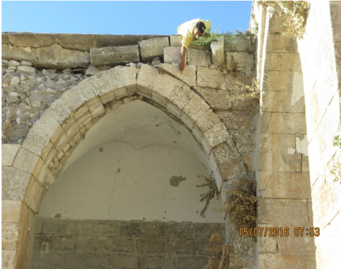
Labelling weak and unstable stone for removal (continued)
