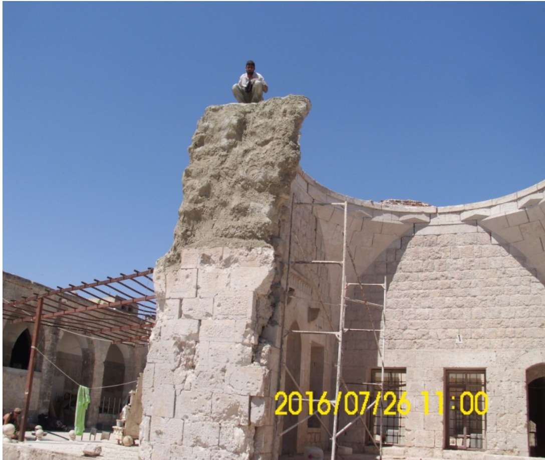
Damaged areas patched with a cement mortar
