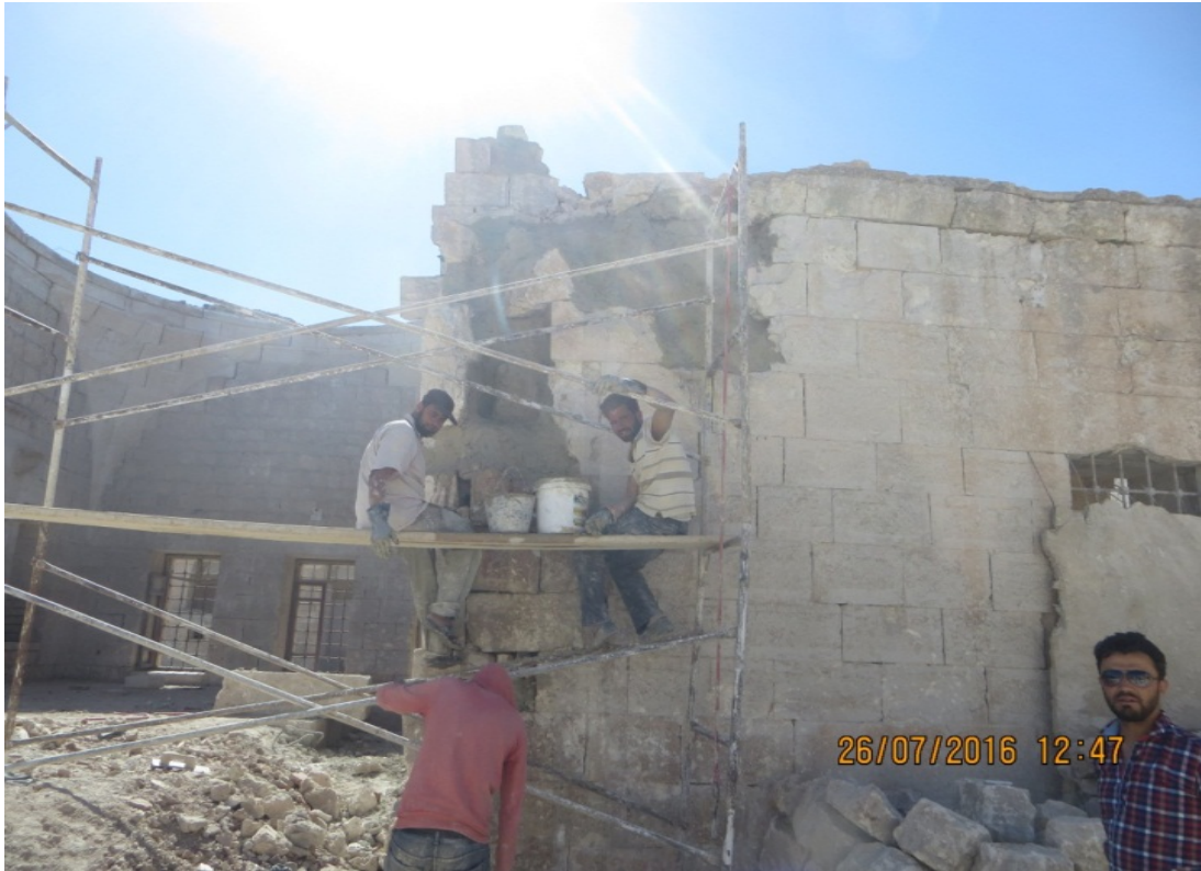
Repairing and stabilizing walls using a cement mortar
