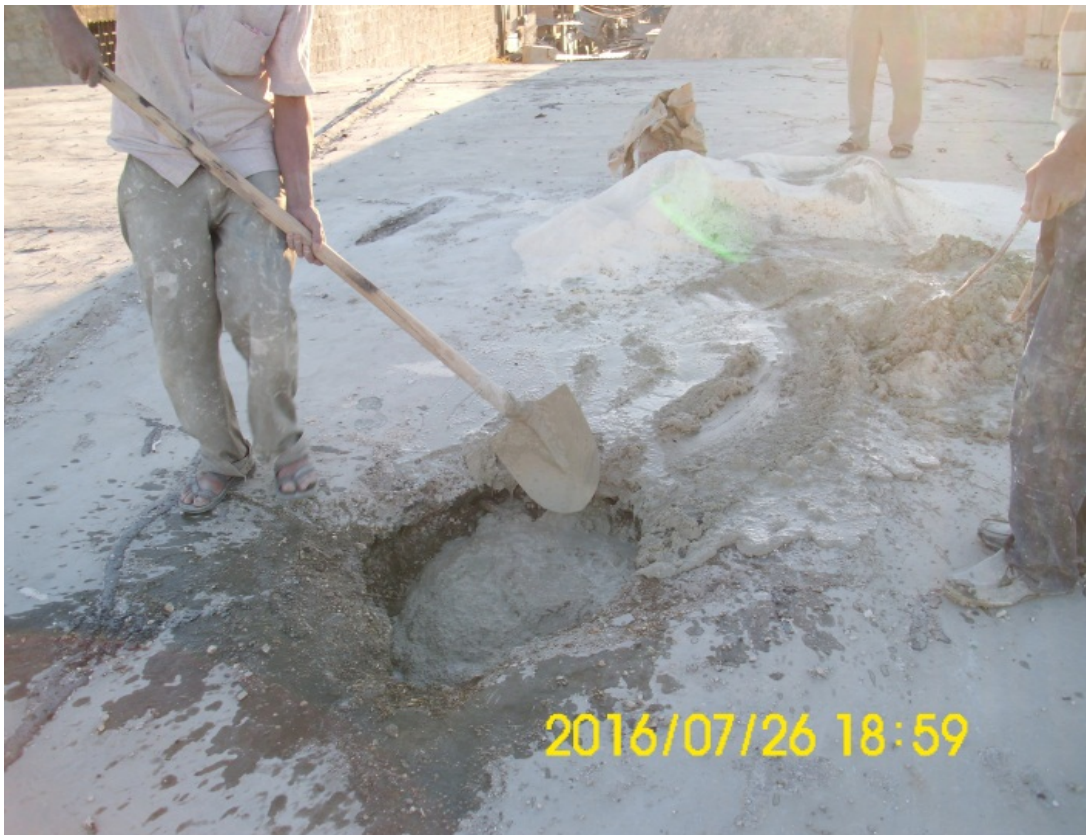
Repairing holes in the roof
