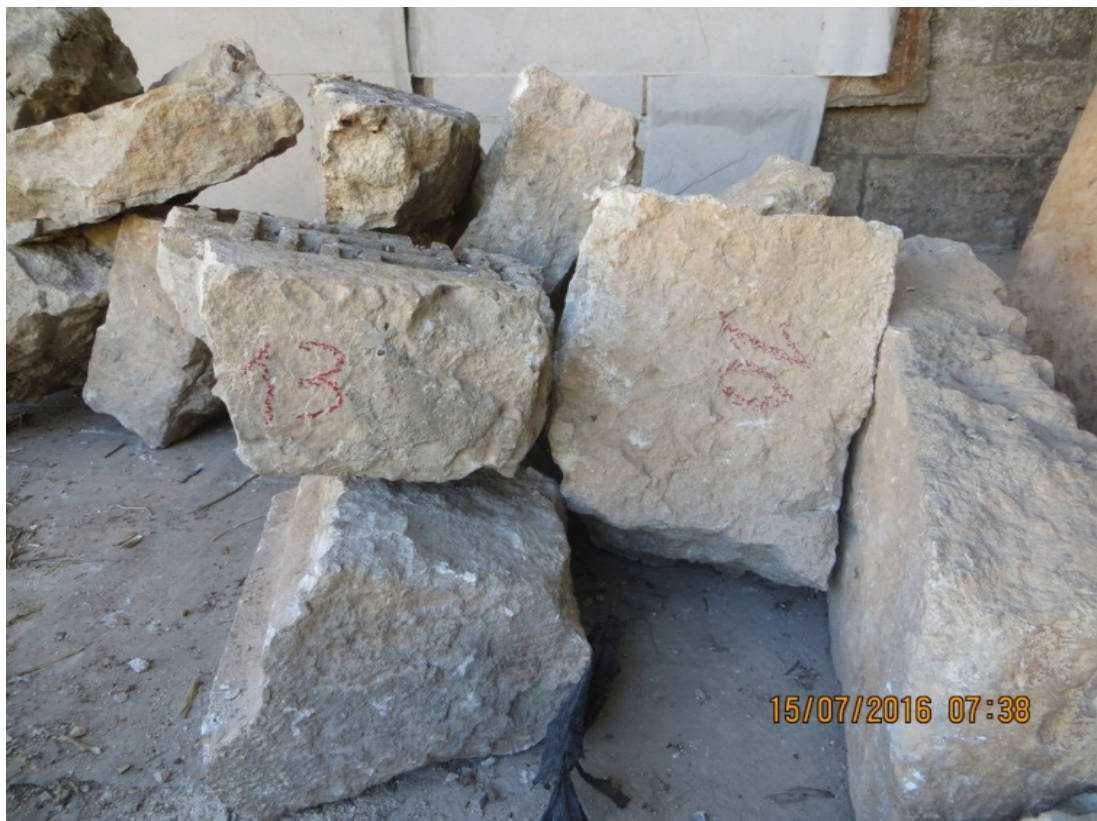
Labelling stone masonry
