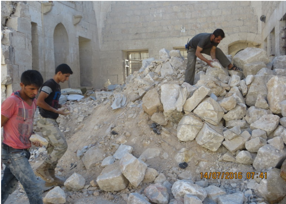
Sorting and removal of stone and rubble (continued)
