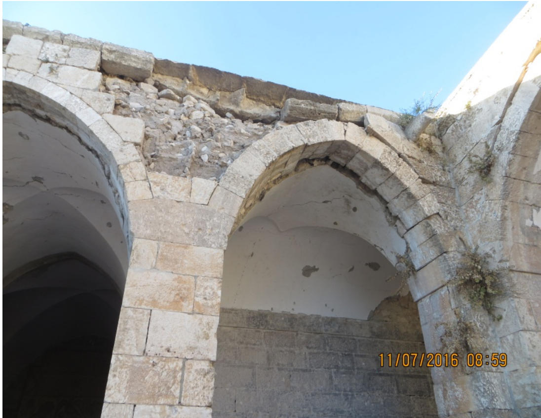
Damage to the arches and the ceiling in the east gallery
