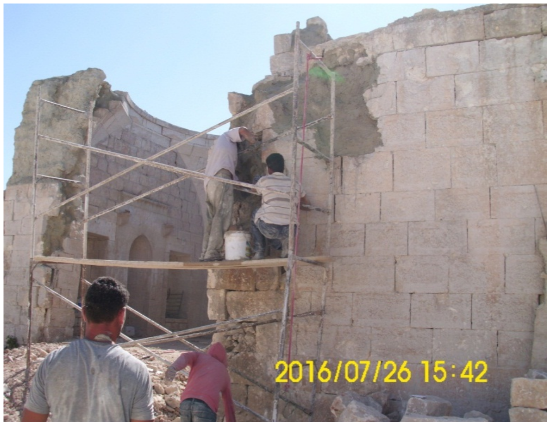
Repairing and stabilizing walls using a cement mortar
