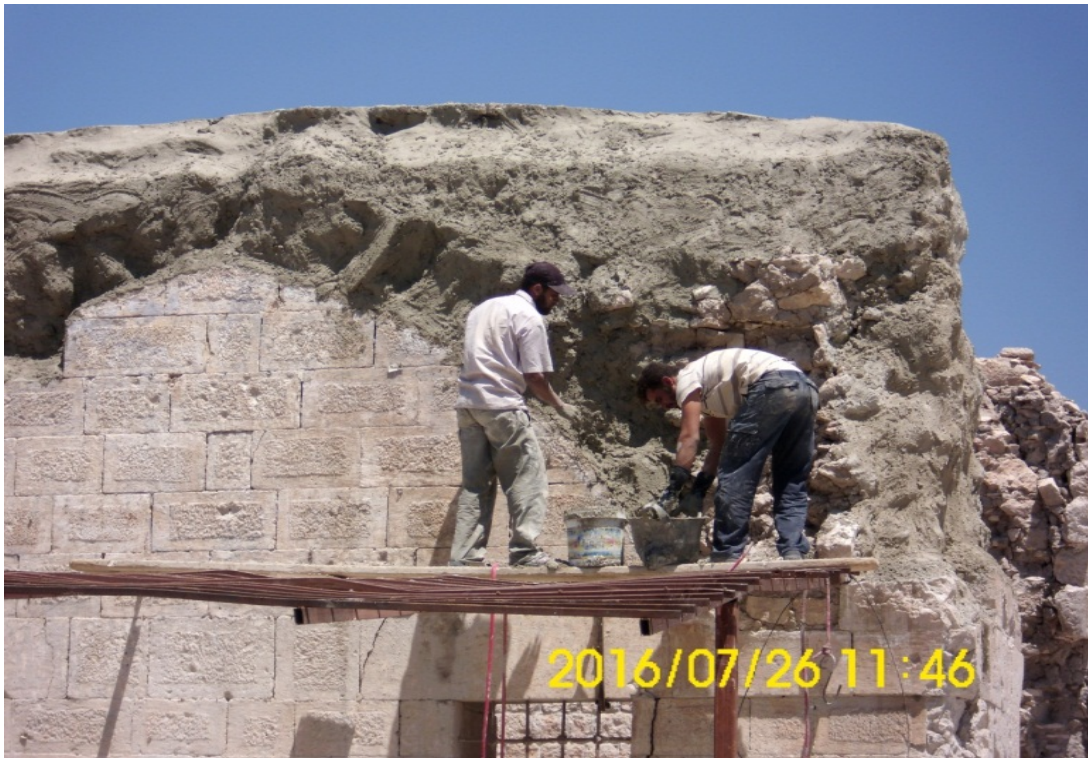
Damaged areas patched with a cement mortar
