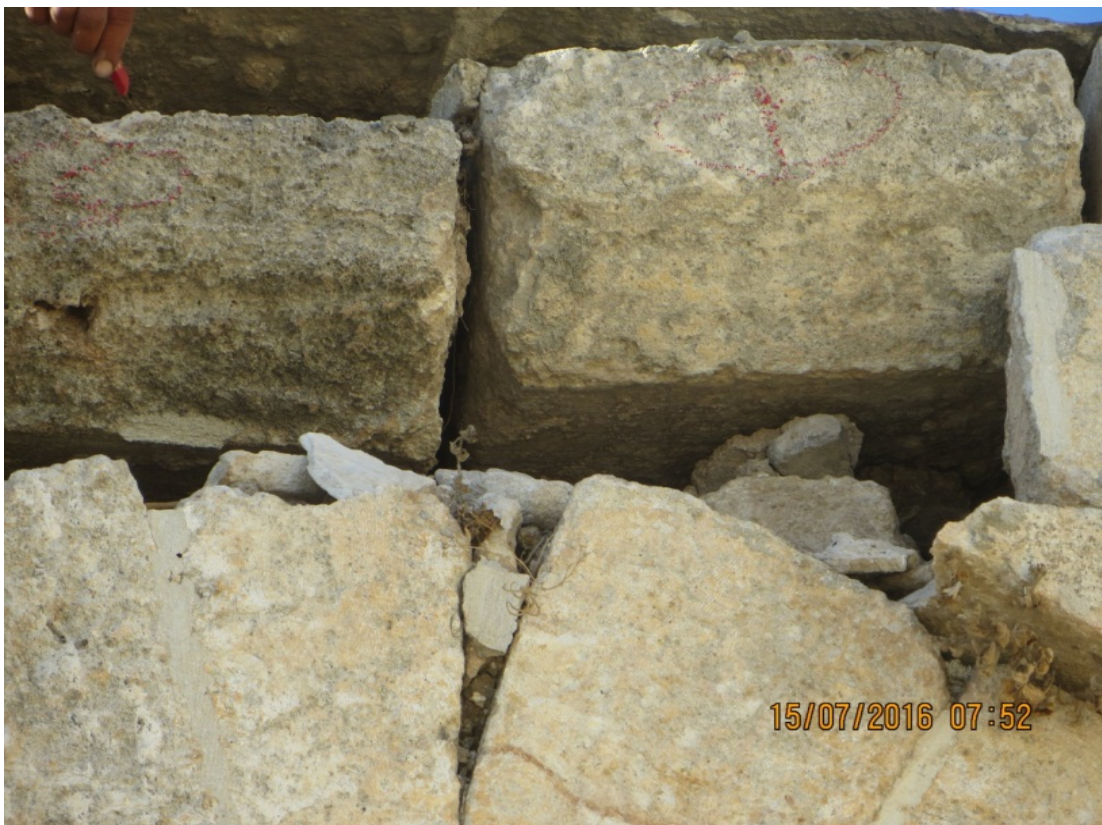
Labelling weak and unstable stone masonry for removal (continued)
