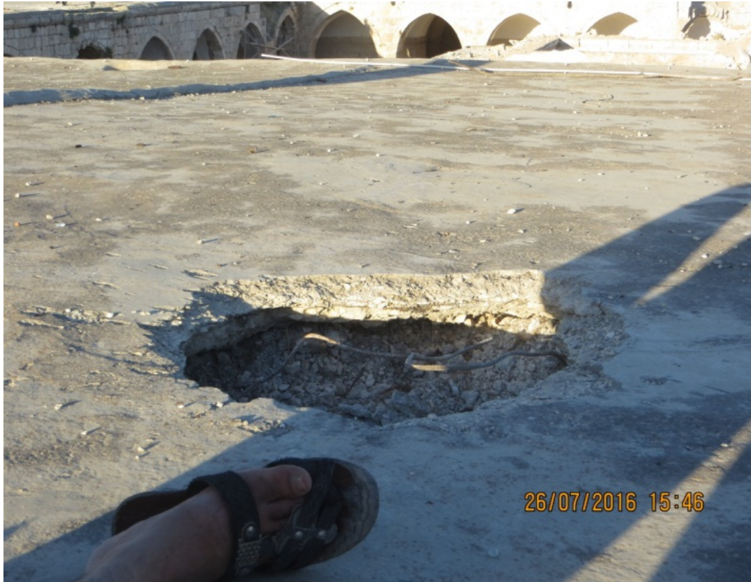
Repairing holes in the roof
