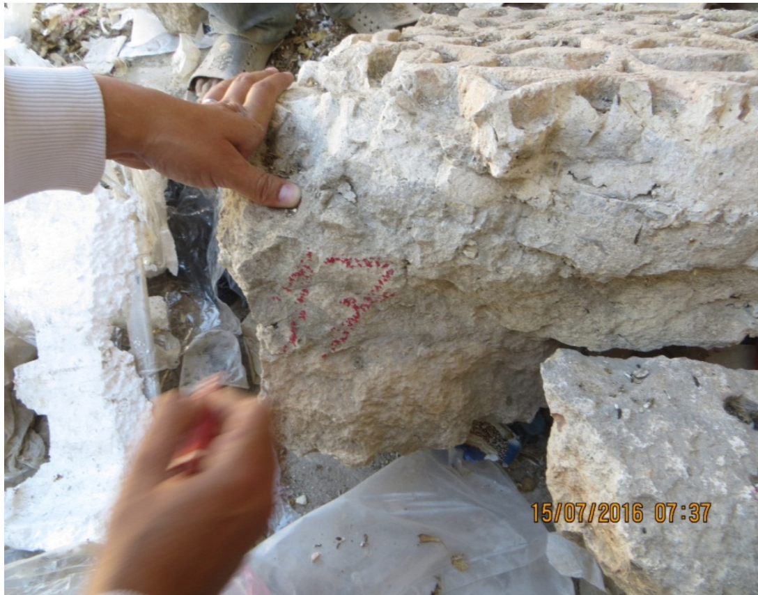
Labelling stone masonry
