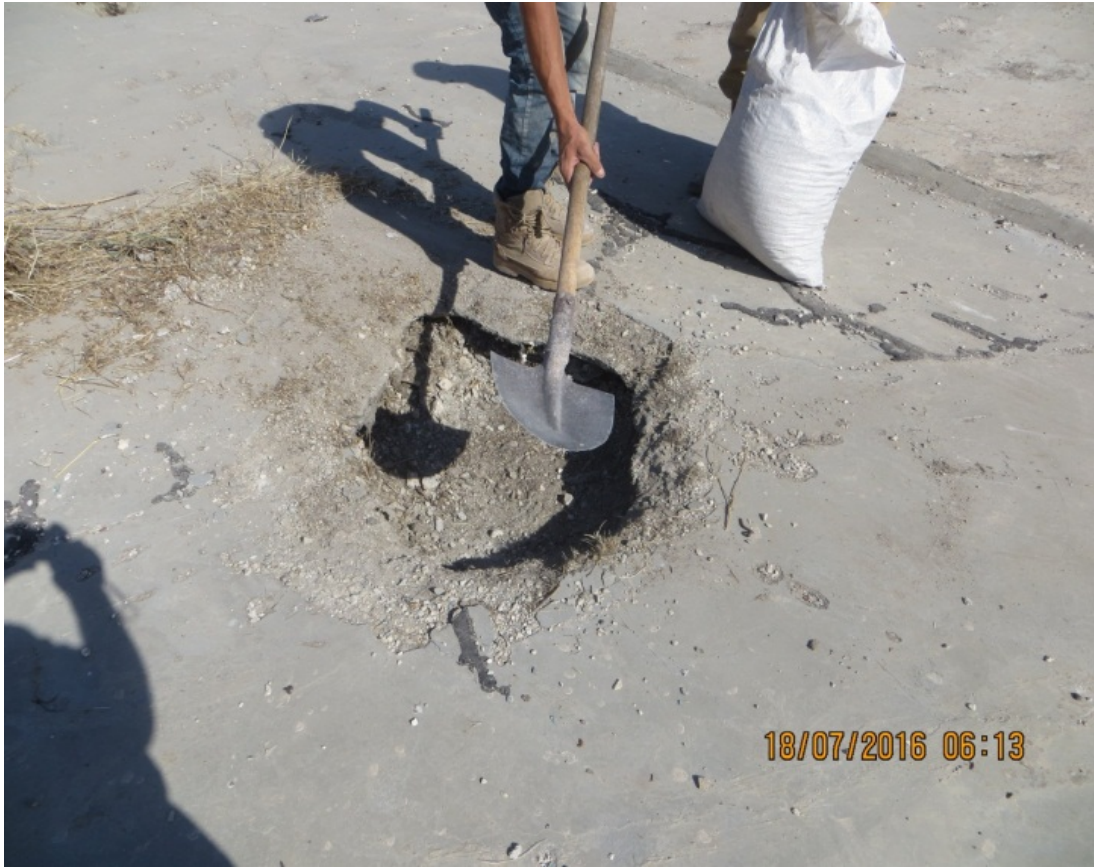
Repairing damaged area on the roof
