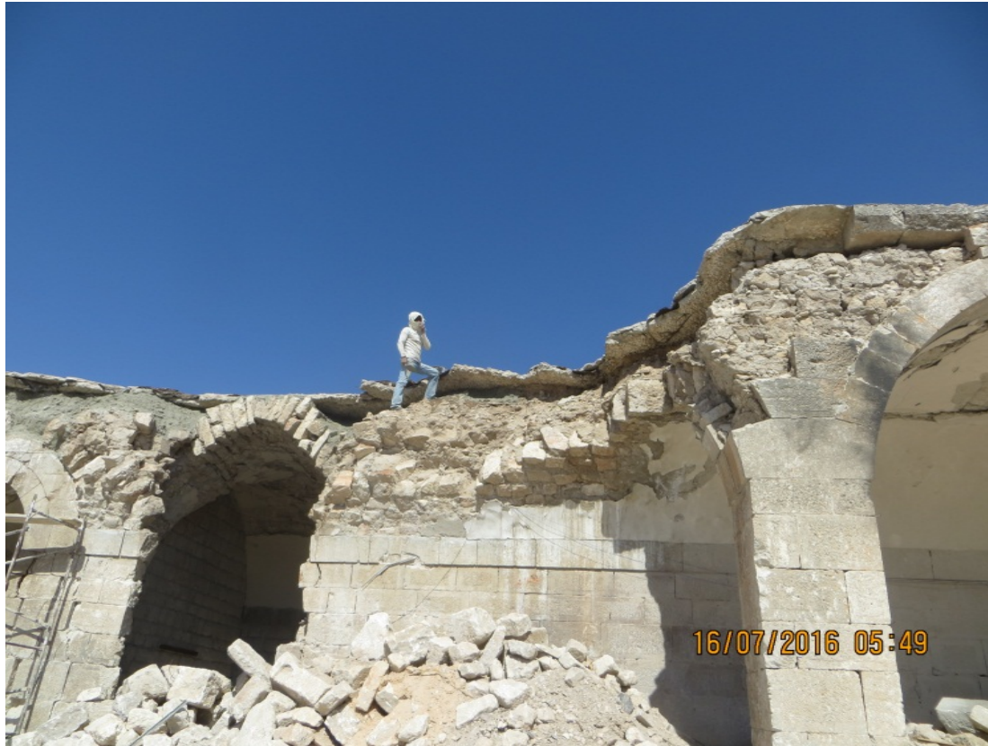
Loose masonry and exposed roof/wall fill
