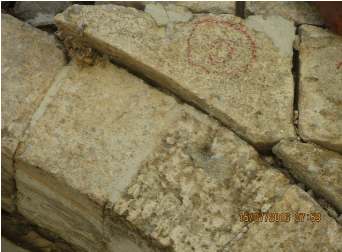
Labelling weak and unstable stone for removal (continued)
