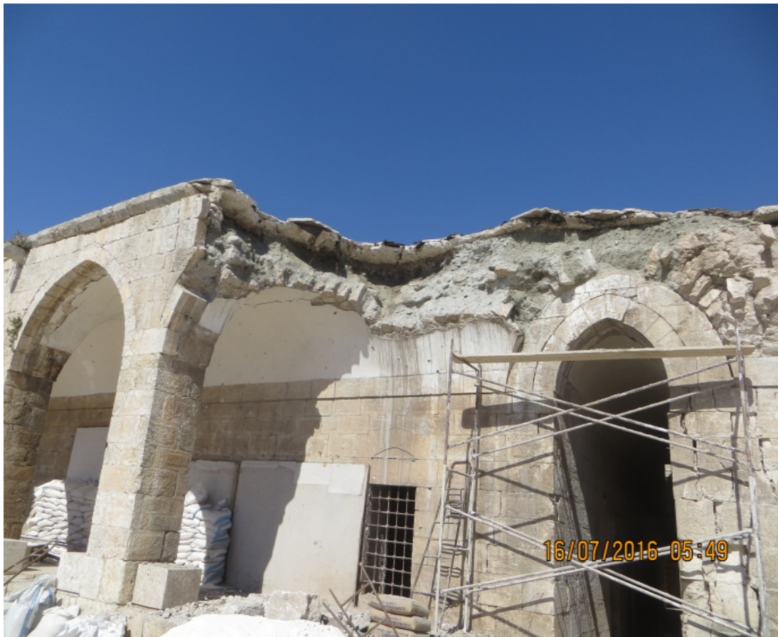
Loose masonry and exposed roof/wall fill (continued)
