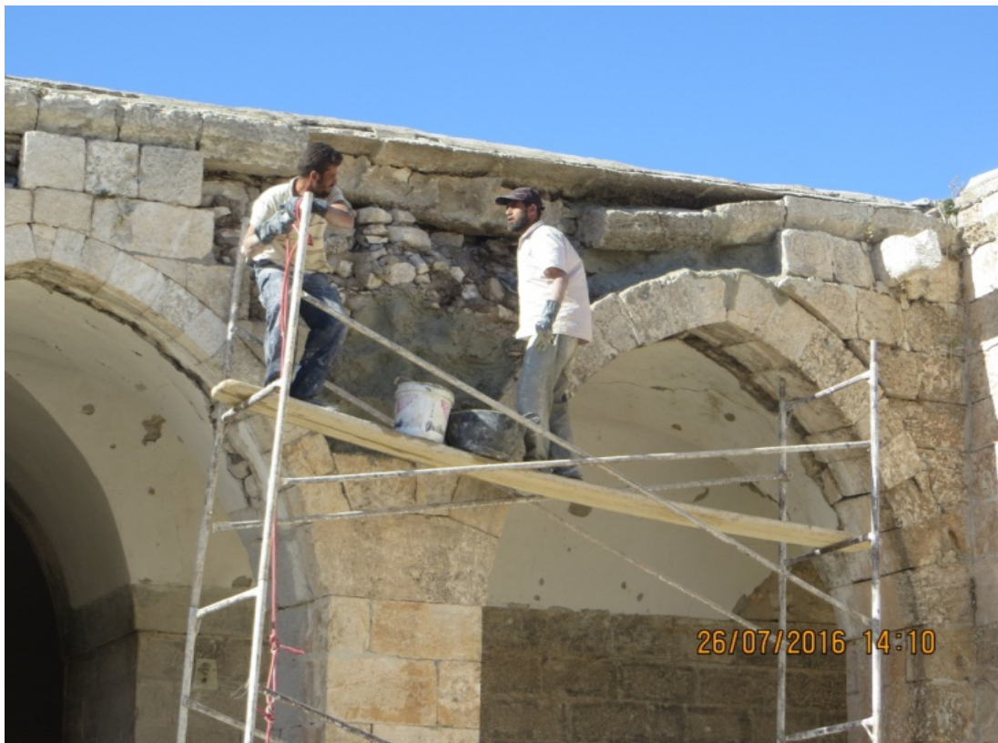
Patching the exposed damage area around the supporting arch with cement mortar
