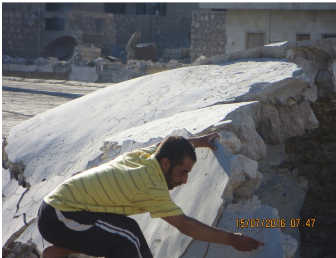
Labeling stones in the Tekkiye prior to removal
