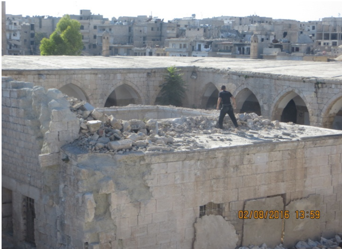
Gradual removal of the Tekkiye stone masonry
