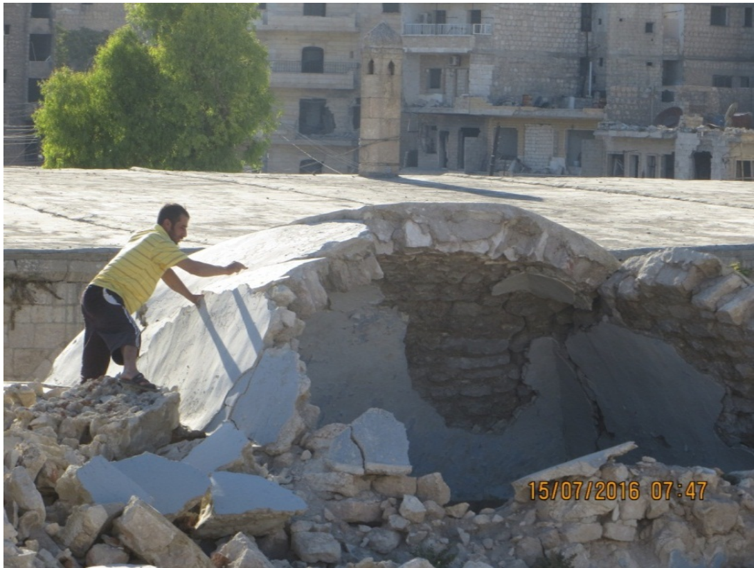
Labeling stones in the Tekkiye prior to removal
