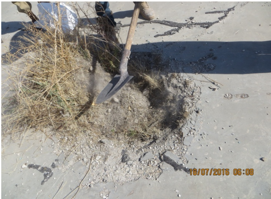
Cleaning roof and preparing it for resurfacing and repair
