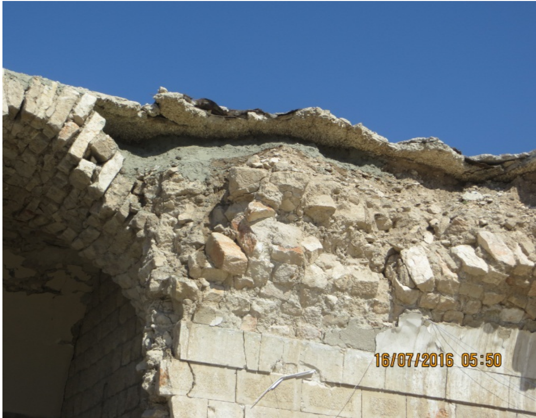
Loose masonry and exposed roof/wall fill (continued)
