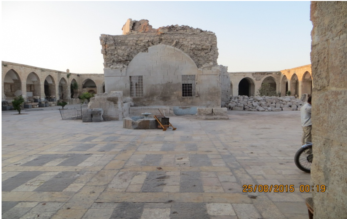
South side of the mosque (facing north) prior to removal of the dome.
