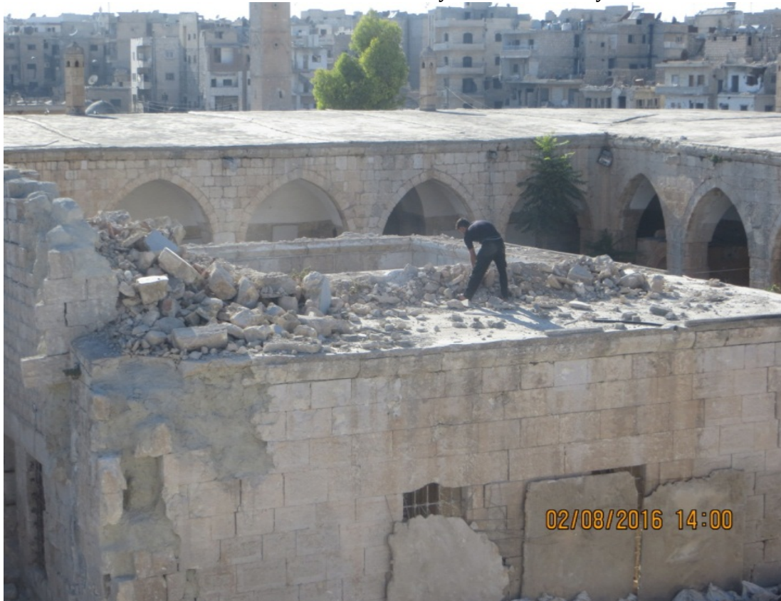
Gradual removal of the Tekkiye stone masonry
