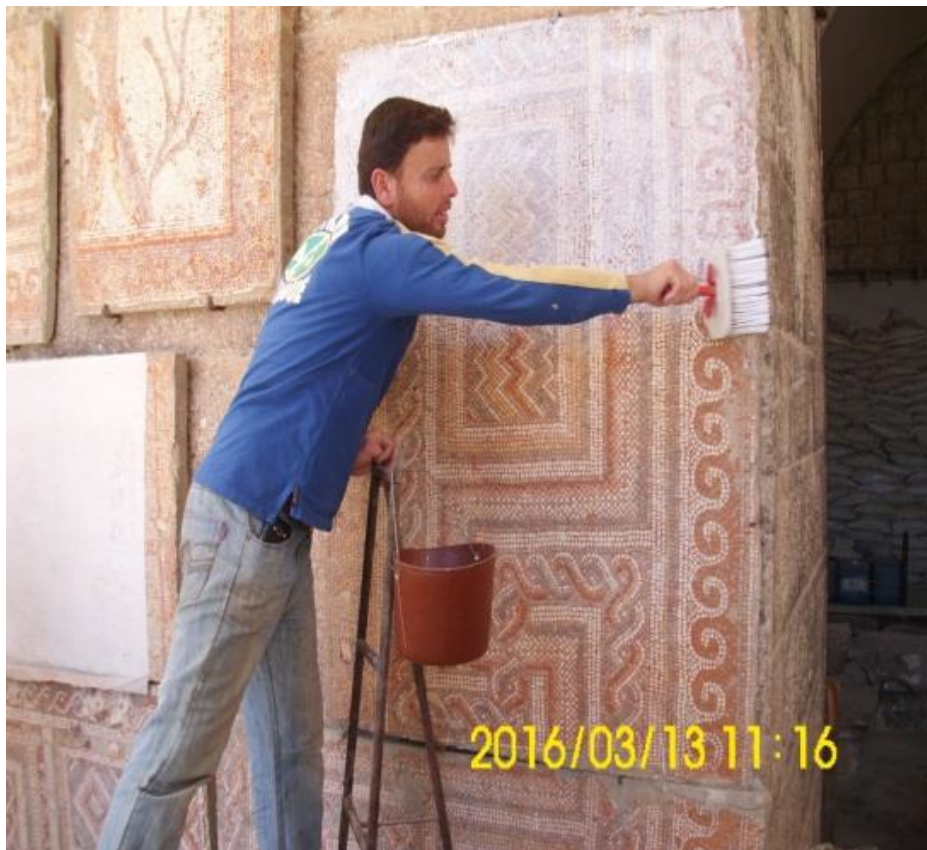
Applying white glue in preparation for laying on the TYVEK
