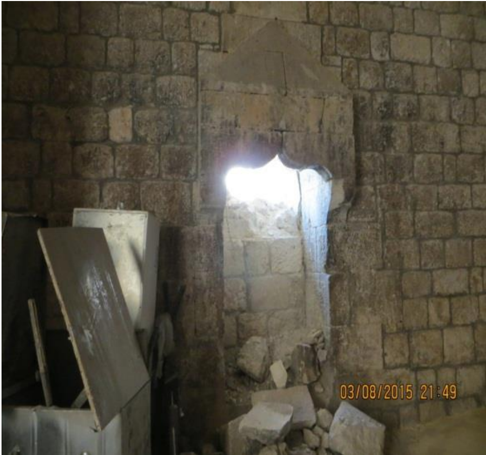
Repairing damage caused by a mortar shell
