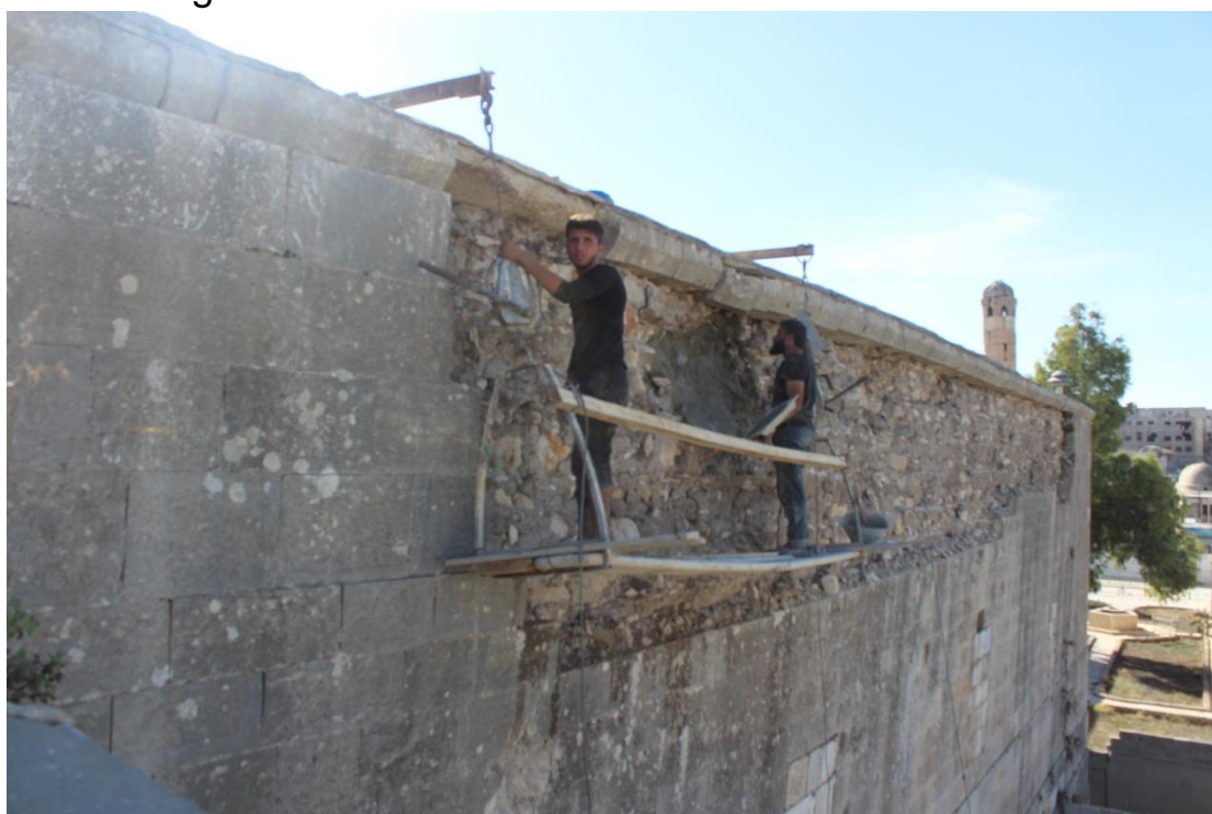
Reinforcing the wall from the north side
