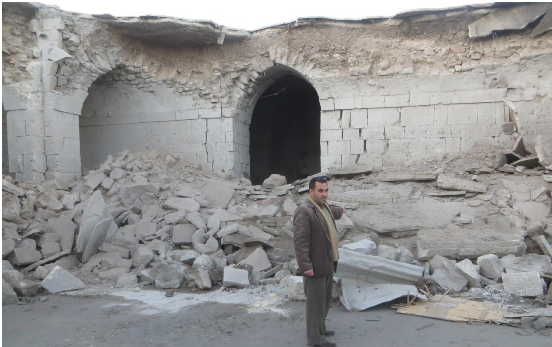
Documenting the damage
