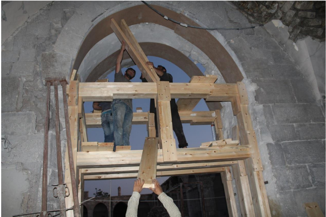
6-Wooden beams being positioned to provide support for the arch.
