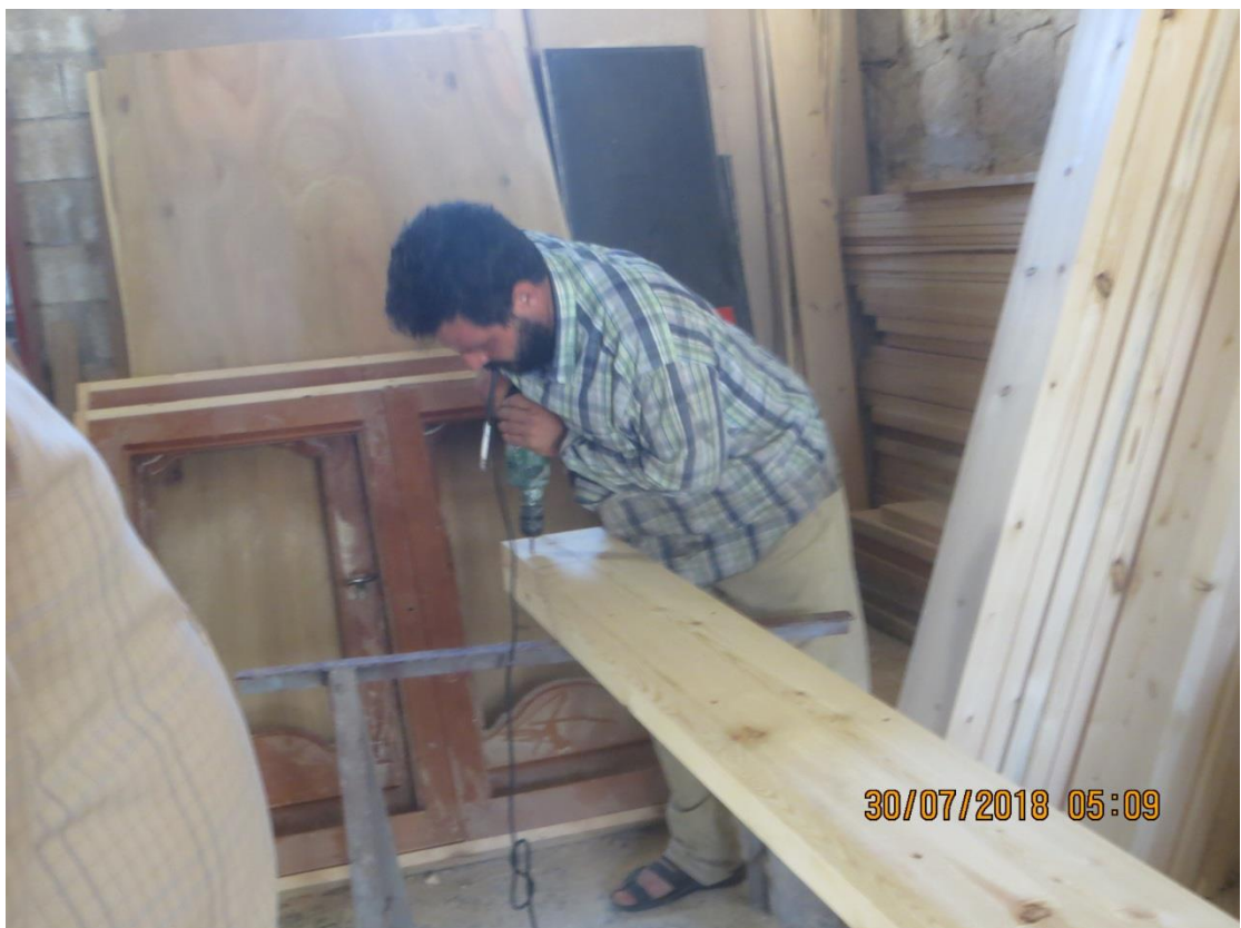
2- Assembling the support beams using glue and screws.
