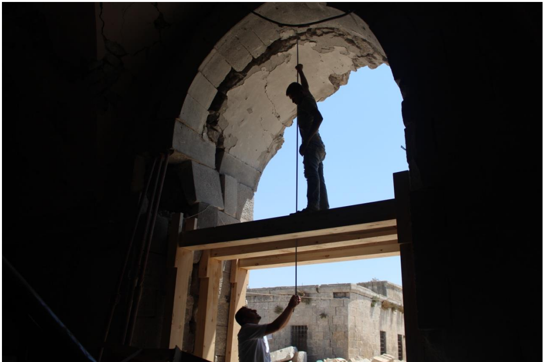
5- Positioning the wooden support beams in place.
