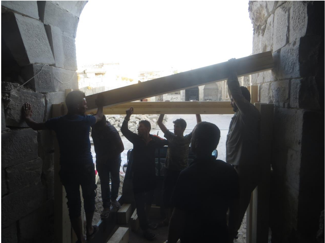
5- Positioning the wooden support beams in place.
