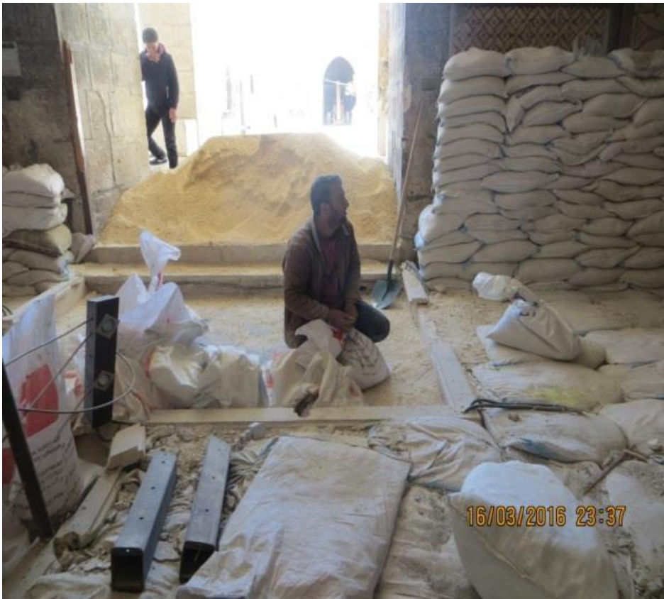
Preparing and filling sandbags
