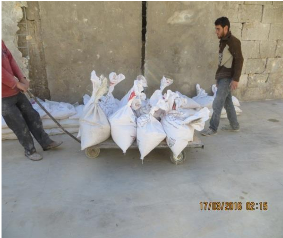
Stacking sandbags against external walls in courtyard for protection
