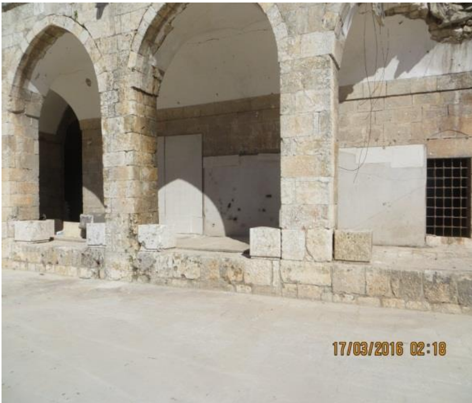
Mosaics covered in TYVEK and ready for removal
