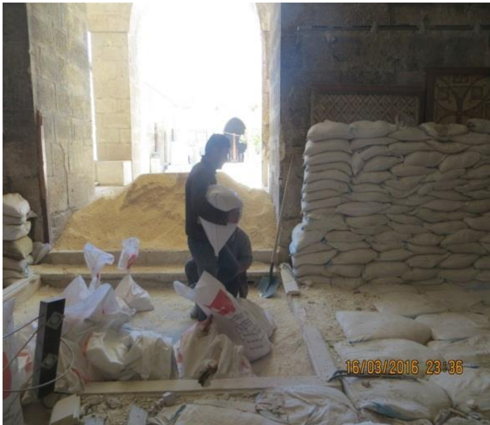
Stacking sandbags against the mosaics for protection
