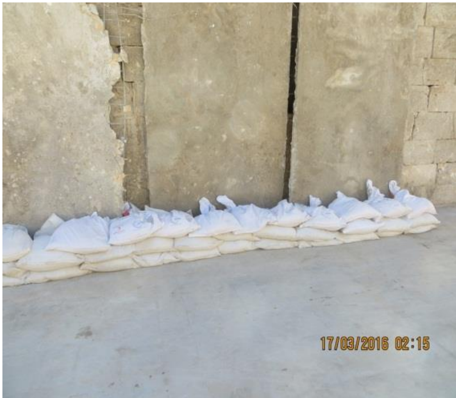
Stacking sandbags against external walls
