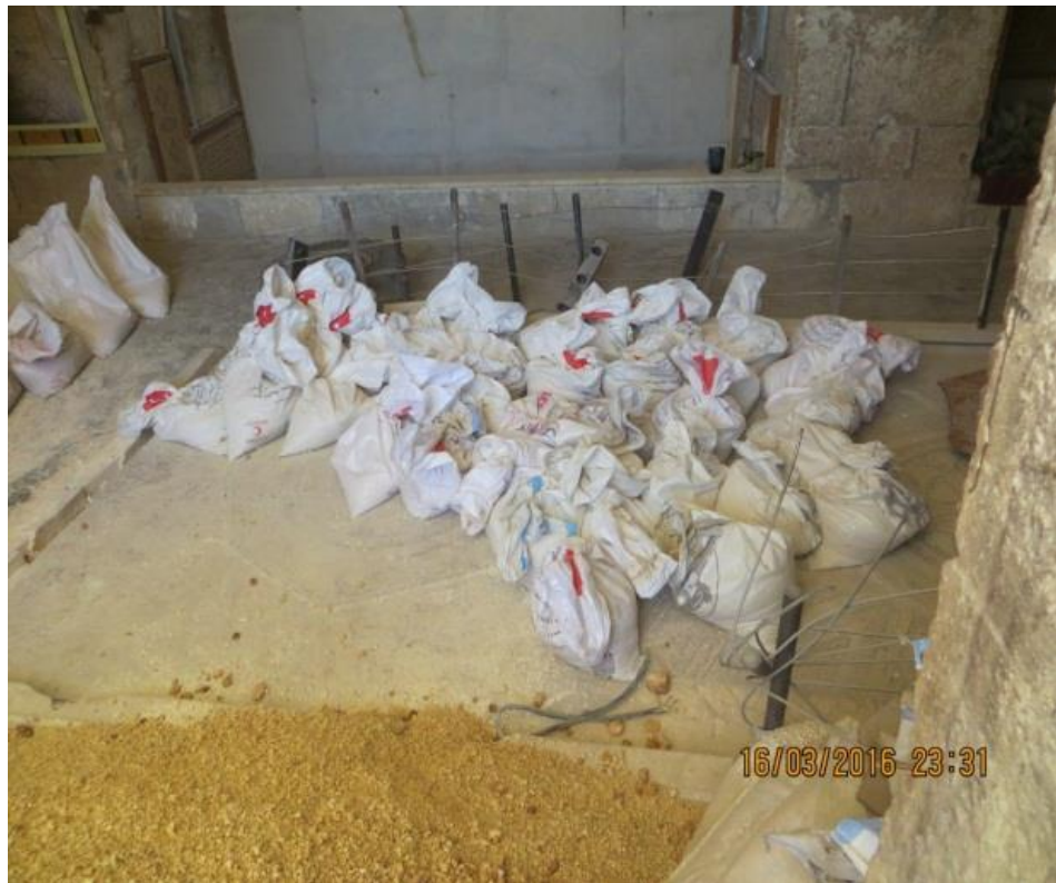
Preparing sandbags to lay against the mosaics.
