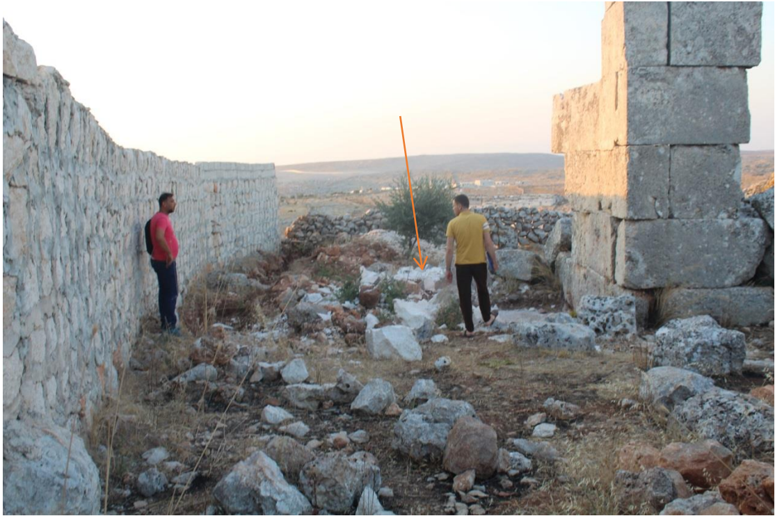
Damages and vandalism
