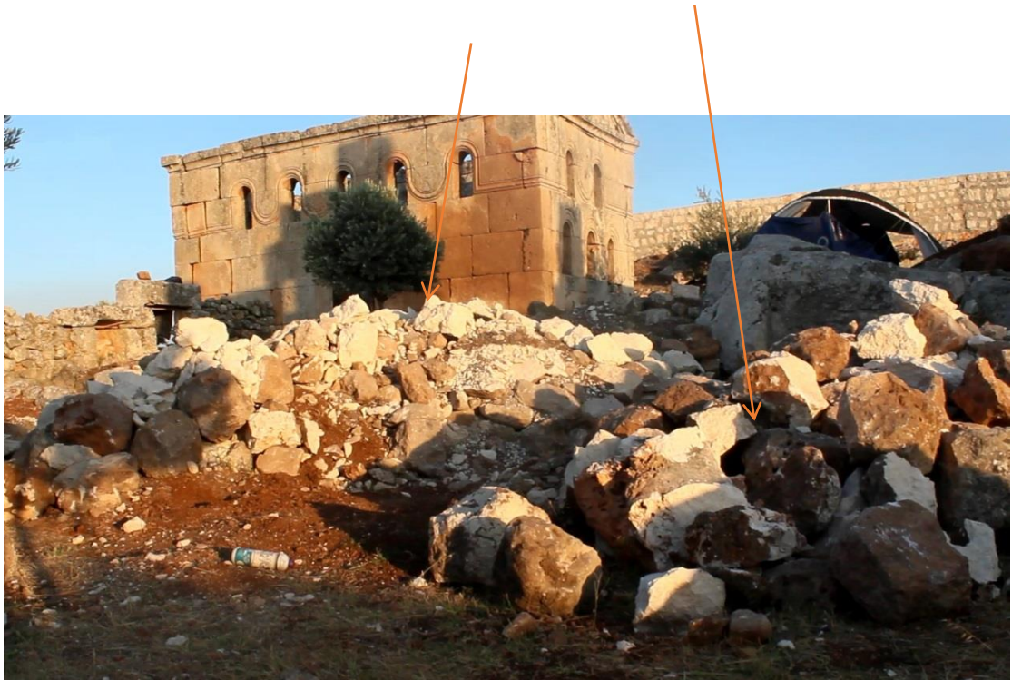
Damage and vandalism
