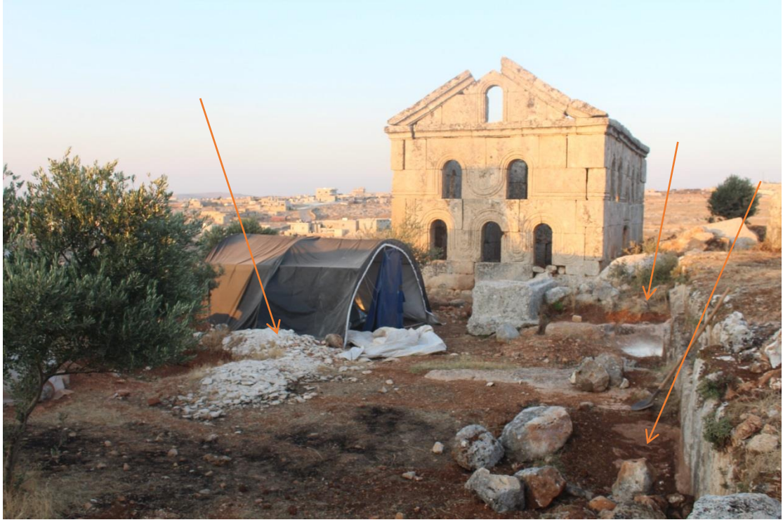
Damage caused by breaking up masonry
